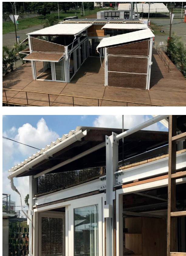
Figure 10 | Mobile system roof and flexible water recollection solution. Source: PEI Team.
