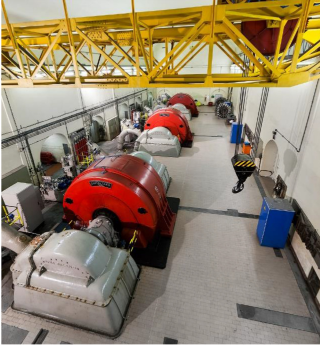
Fig. 1. A picture of the Signayes Hydropower Plant from C.V.A. S.p.A.
