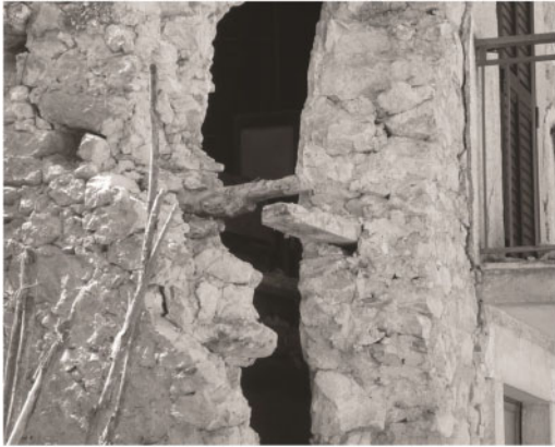
Figure 3. Villa S. Angelo (AQ), wooden radiciamenti placed in the thickness of corner walls.
