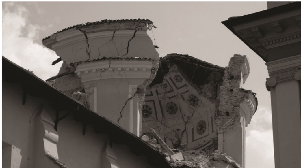
Figure 1. L'Aquila, chiesa delle Anime Sante, three courses of wooden radiciamenti in the drum of the dome.
