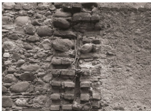
Figure 10. Montalenghe (TO), metal anchor recessed in the masonry toothing revealing the presence of a metal tie-rod in the half-width of the back transverse wall.
