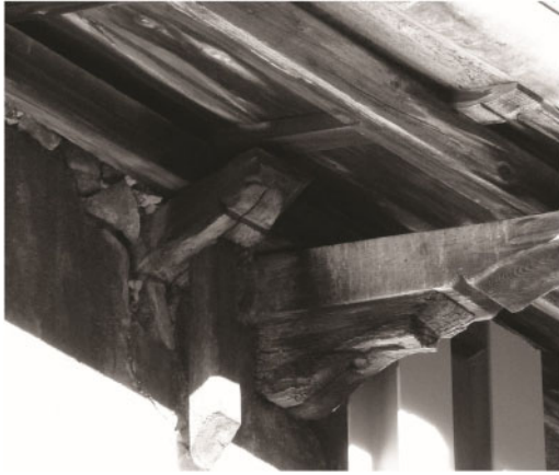
Figure 6. Detail of a wooden anchor connecting the roof trusses to the external wall.
