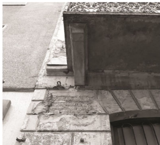
Figure 11. Turin, the closeness to the façade edge of the metal anchor reveals that the corresponding tie-rod is embedded in the orthogonal wall.
