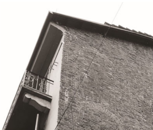
Figure 9. Turin, anchors of façade's metal radiciamenti emerging from recesses housed in the transverse wall.
