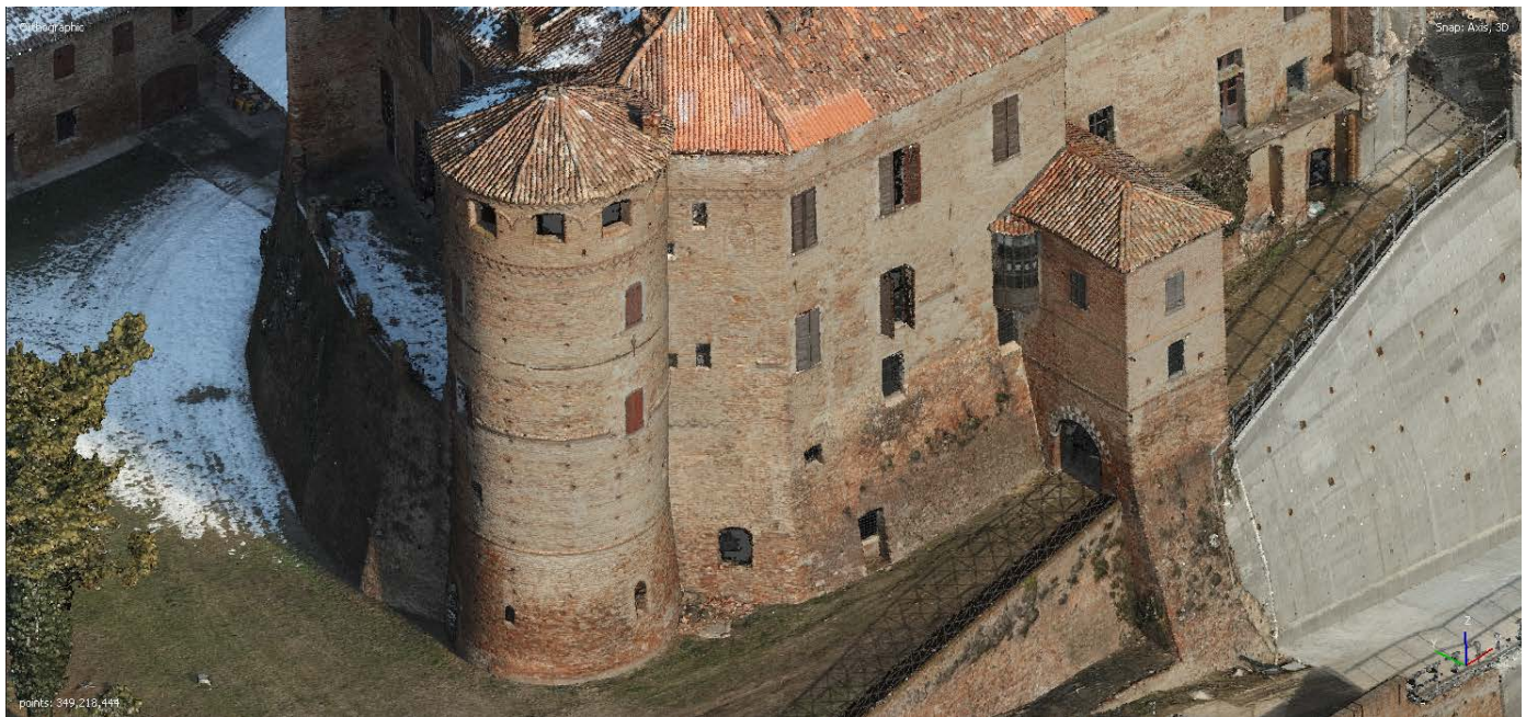
Figure 8. Photogrammetric output via Agisoft Metashape: detail on the east–west side of the castle and the circular tower (point dimension 1 pixel).
