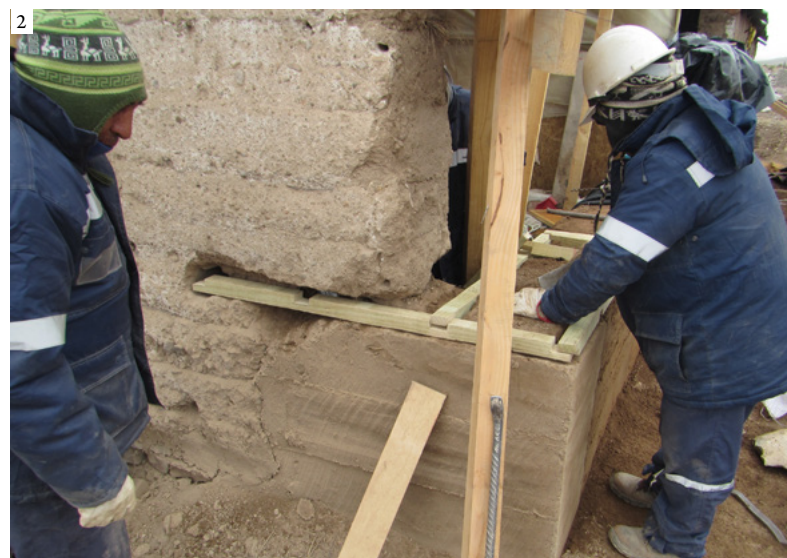
2: Wooden reinforcement of a rammed-earth wall
