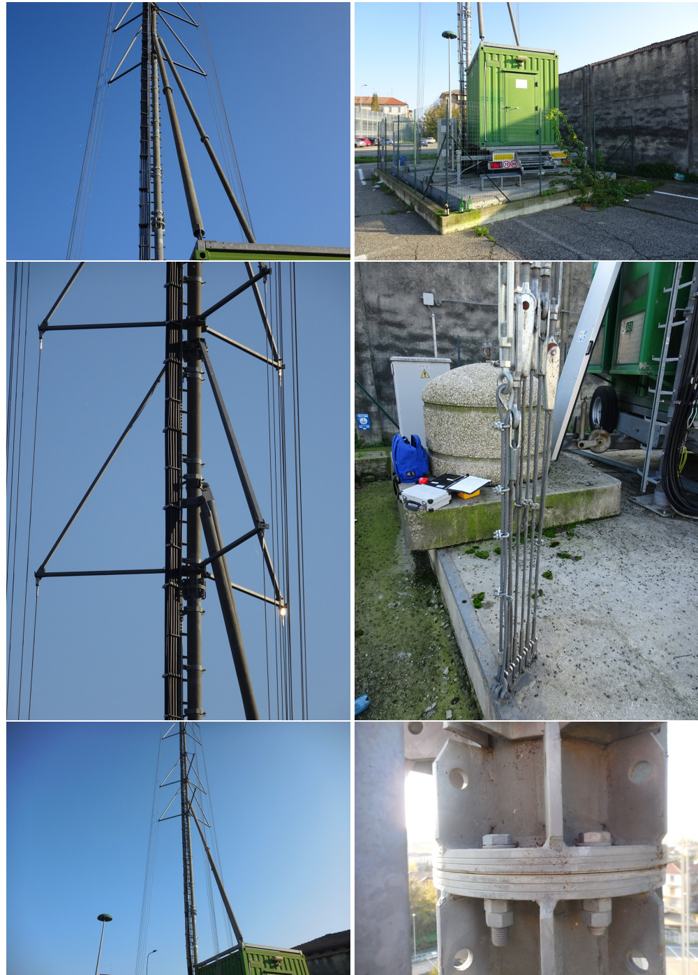
Figure 2. Pictures and details of the considered structure.
