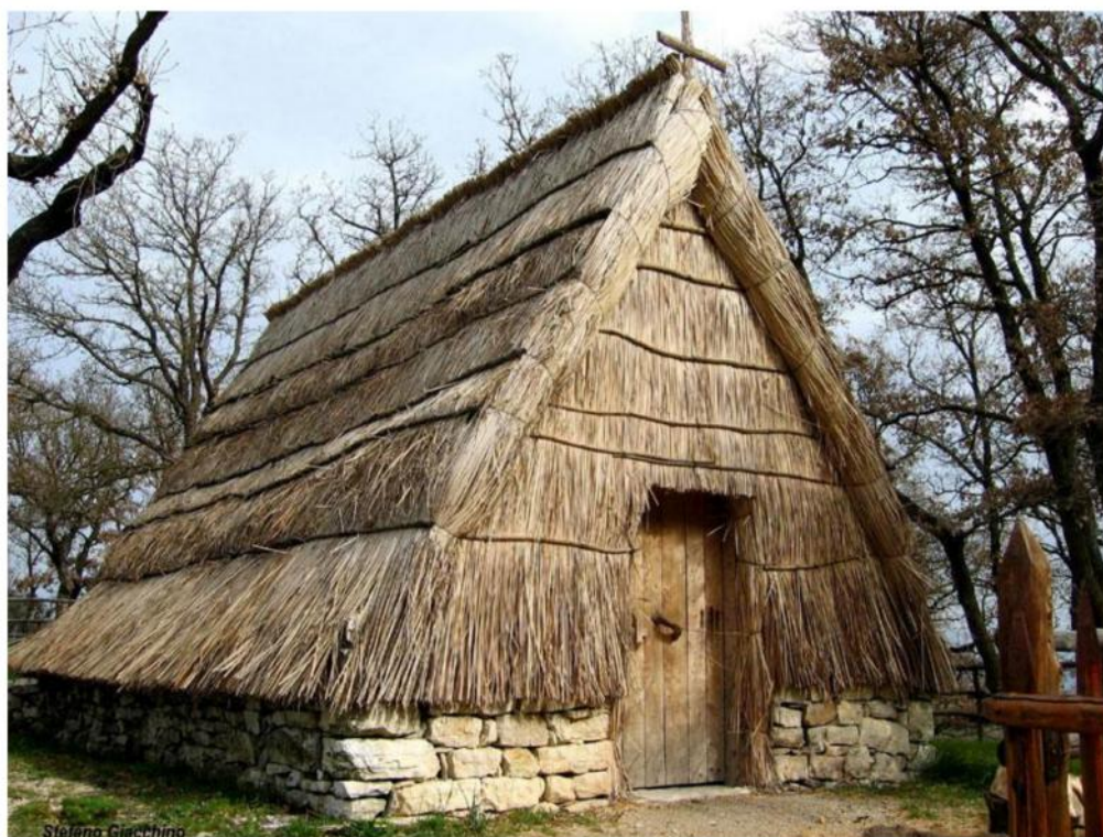
Figure 1. Example of Pagliaru Longu , Monte Carcaci, Sicily. This type of pagliaru is distinguished by a rectangular base. Its maximum size was around 5 m 2 (54 ft 2 ). Photo credit: Stefano Giacchino [31].
