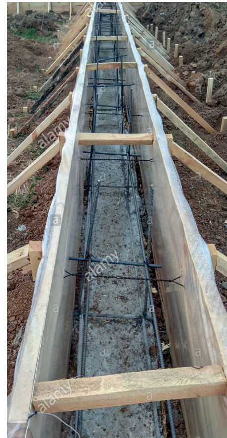
Cassero in legno da https://www.alamy.it/cassero-in-legno-cemento-fondazione-striscio-per-un-cottage-2018-image219021678.html
