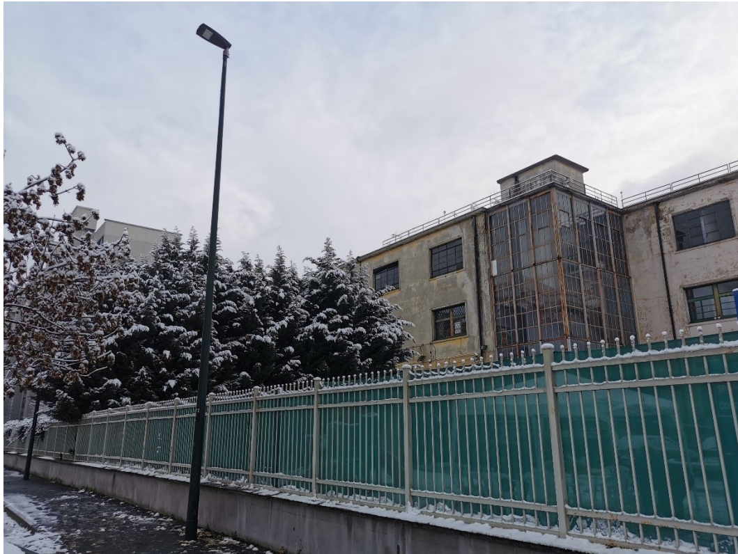
Figure 7 A view of the dormitory from the street
