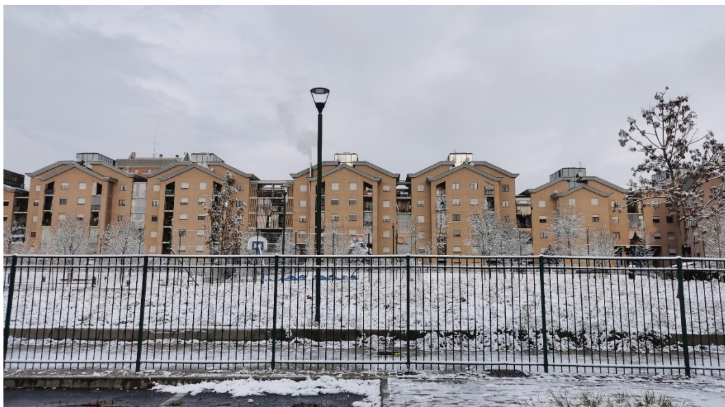
Figure 6 Front view of part of the public housing complex in front of the centre
