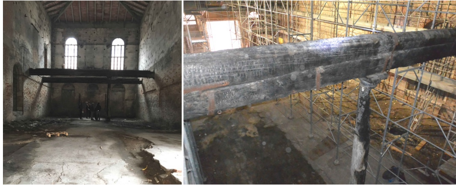
Fig. 5 Interior view of the Sala d'Armi “E” (left), detail of the burned wooden beam with wooden column (right). (Photo D. Ferrante, 2019)
