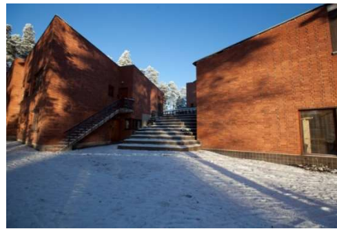
Fig. 5-13 The design of the entrance is influenced by multiple, humanity and adaptability (Chard, 2014)
