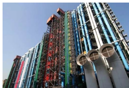
Fig.2-16 Centre Pompidou, 1977 (Kranendonk, n.d.)
