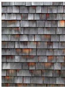
Fig. 3-4 The hardened wood façade was adopted in Saint Benedict Chape (Lin, 2017)
