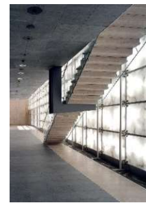
Fig. 3-5 A translucent stone facade was adopted in Deutsche Bundesbank (Bitter, n.d.)
