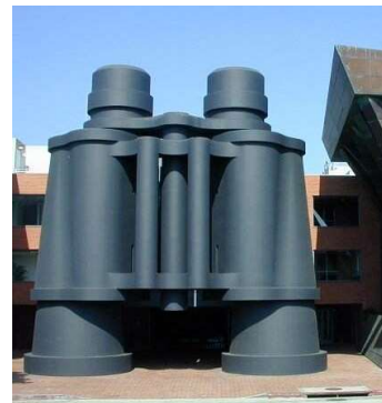
Fig.2-14 Chiat/Day building (n.d.)
