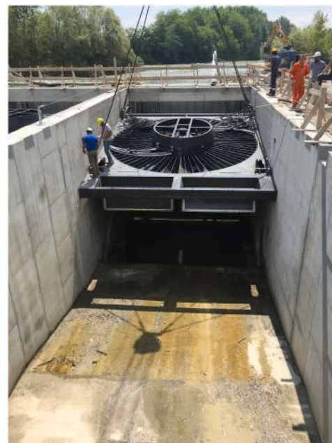
(b) Installation on the movable guide
