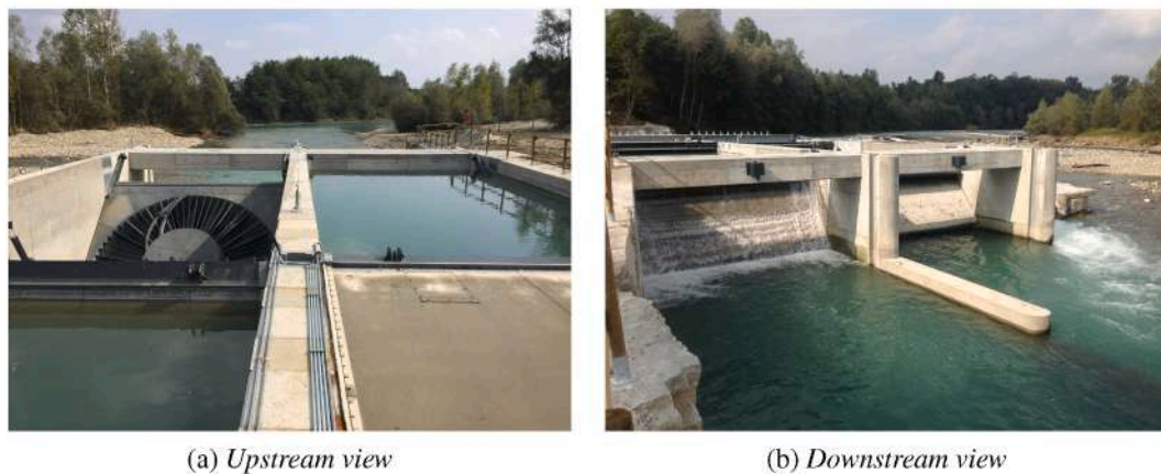
Fig. 3. VLHT installation in a canal, Mazzè, Italy. 2.60 m head, two VLHTs for a total of 54.2 m 3 /s, 5 m diameter each, 1000 kW of installed capacity and 25 m long derivation canal. Photo Courtesy Geasiste.
