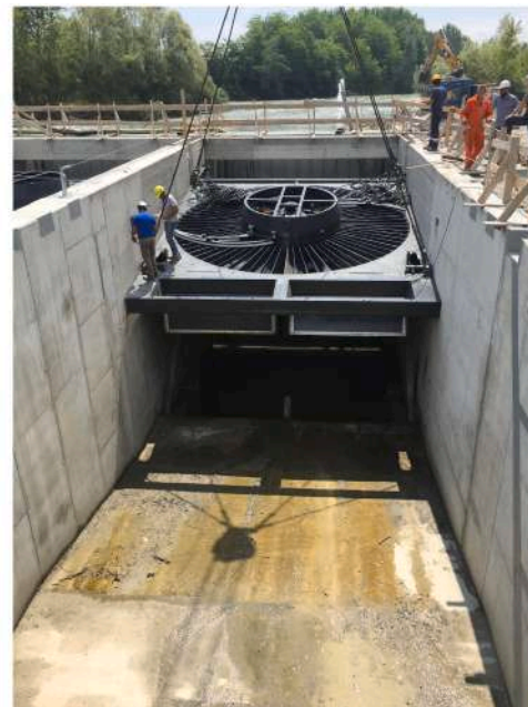
(b) Installation on the movable guide
