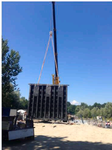
(a) Transport and uplift by crane
