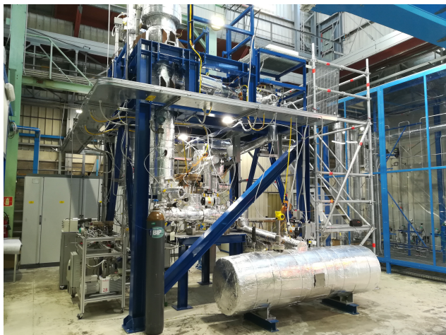
Figure 2: TRIEX-II LiPb facility.
