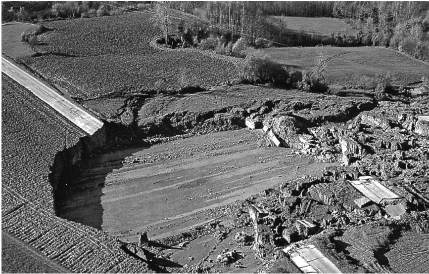
Fig. 6 – Planar landslide immediately after failure. Typical landslide body displaced by a planar sliding mechanism (modified by Bottino et al. 2011).
