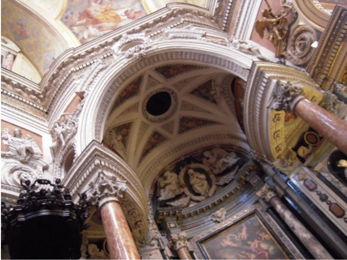
Figure 4: Detail of the vault of the chapel shown in the Figure 3. Let us remark that the chapel has a double vault. We can see a six-pointed star depicted on it with an oculus at the center, a hole which seems totally useless. As told in [26], there is a little secret here. Inside the double vault there is a hidden painting, visible only when the hole in front of the chapel is illuminated by the sun beams. This happens at specific moments of the year and only under good weather conditions.
