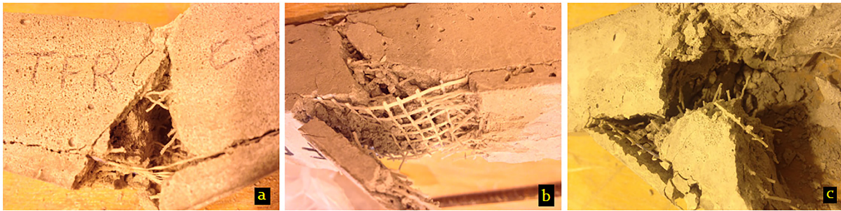
Fig. 21. Photographs at failure of foamed concrete beams cured in cellophane: a) close-up detail at the mid-span beam soffit; b) interaction between short polymer fibers and glass-fiber bi-directional grid reinforcement; c) detail of the rupture zone with concrete detachment.
