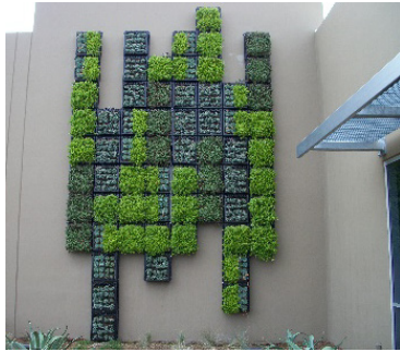
Fig. 3 Panel with soil substrate cells for planting
