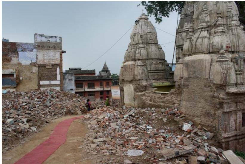
Figure 38 The same area, stretching towards the river, with temples saved from demolitions yet damaged, November 2019. Author's picture.
