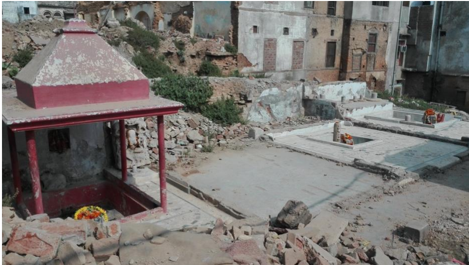
Figure 13 The structures emerging from the demolitions in a spot where I stopped talking with informants during one video-interview.re
