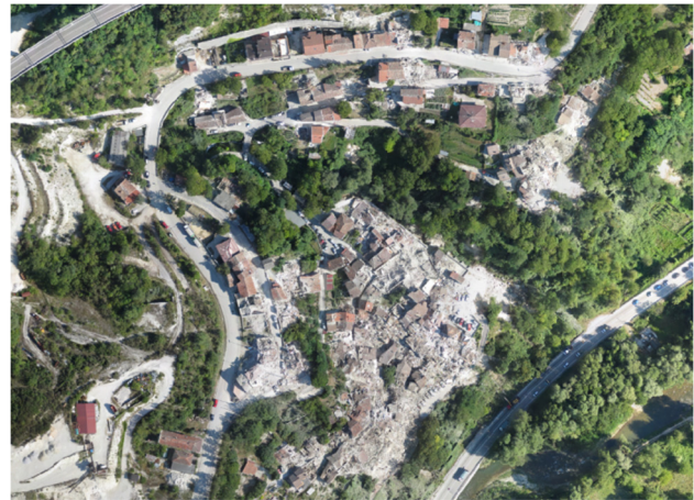
Figure 2. Orthophoto of Pescara del Tronto (Italy) after the 2016 seismic event.
