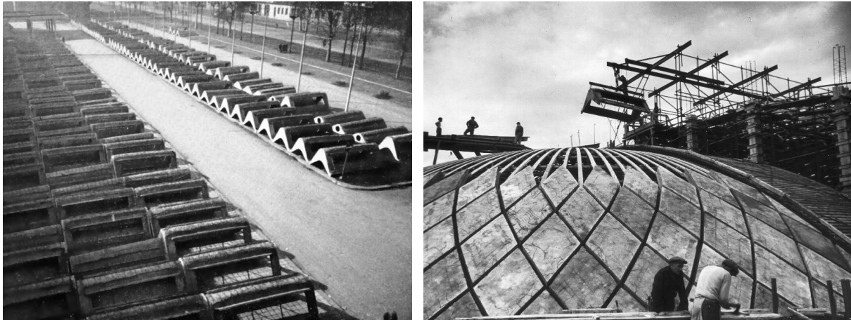
Figure 2: The onsite prefabrication procedure of the undulated ferrocement elements of Hall B and their positioning.
