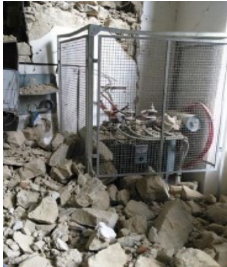
Figure 6-4. MV/LV substation damaged after the 2016 Central Italy earthquake (Rieti, Italy).
