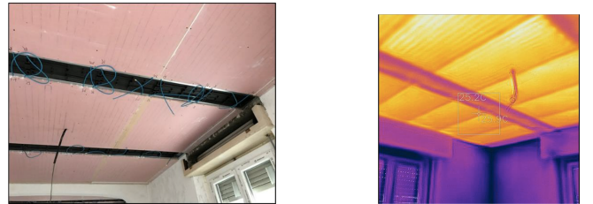
Fig. 1. Installation of the heating system (left) and thermography picture of the panels while working, by means of a thermoscanner (right)
