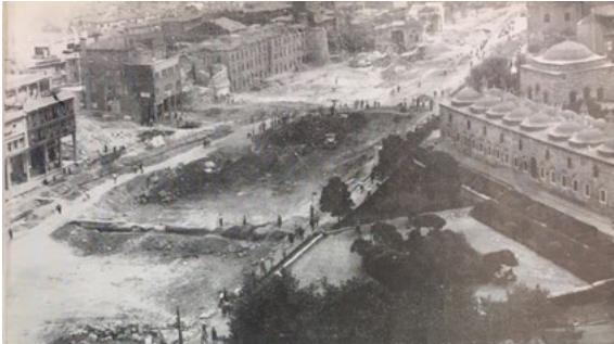
Figure 19. Istanbul. Ordu Avenue during the demolition (from Istanbul'un Kitabı 1957, p. 35).
