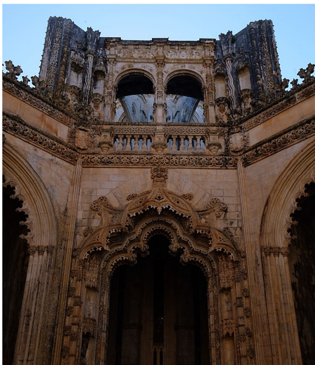
Fig. 1 Facade and ornaments with orange patina at the Imperfect Chapels, Batalha Monastery
