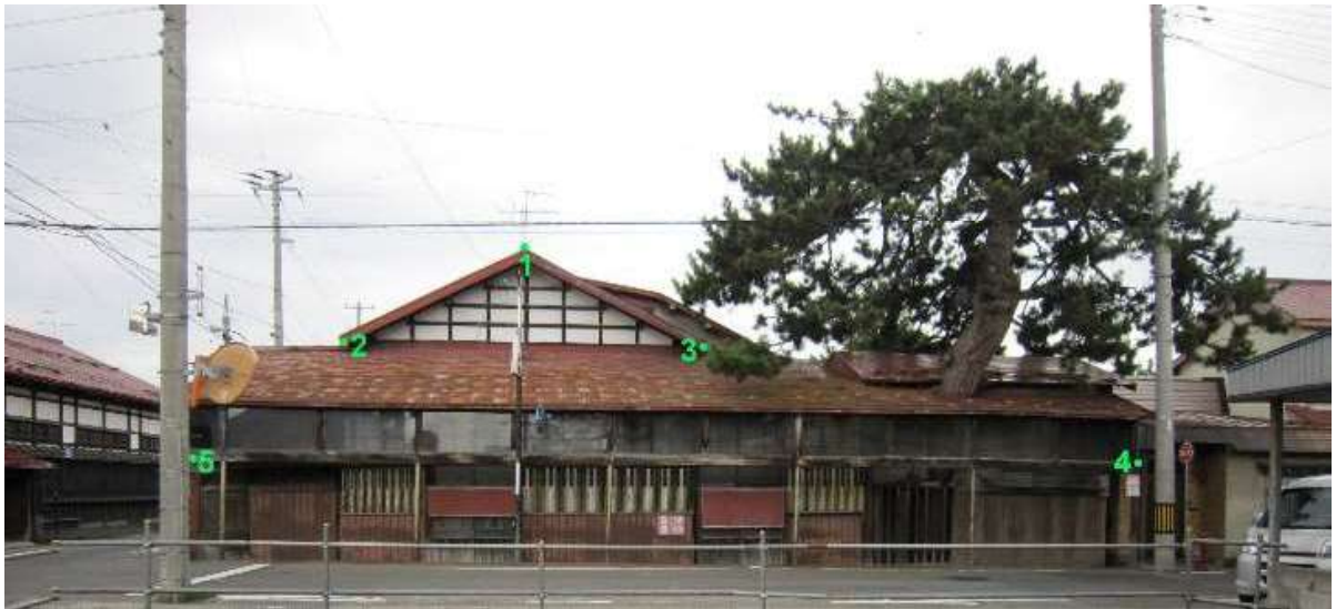
Figure 101. Feature points manually chosen for the Former Matsuno-Yu building.
