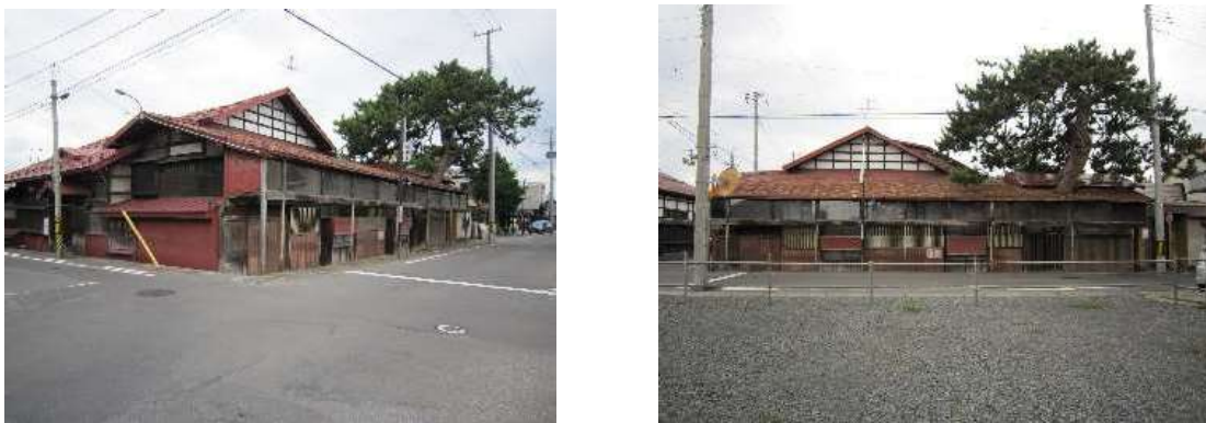
Figure 95. Local archive photographs of the Former Matsuno-Yu building before the restoration in 2013.
