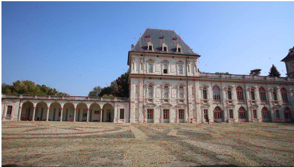
Figure 14. The result of the first step feature detection and extraction of the pipeline. The red points are the Feature Points automatically extracted from the software.
