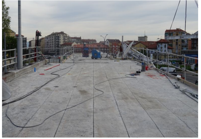
Figure 7. Concrete beam cutting phase.
