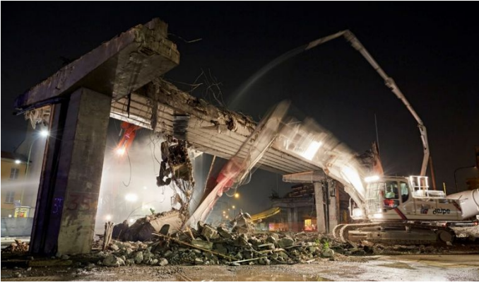
Figure 5. Demolition bridge process using hydraulic pliers.
