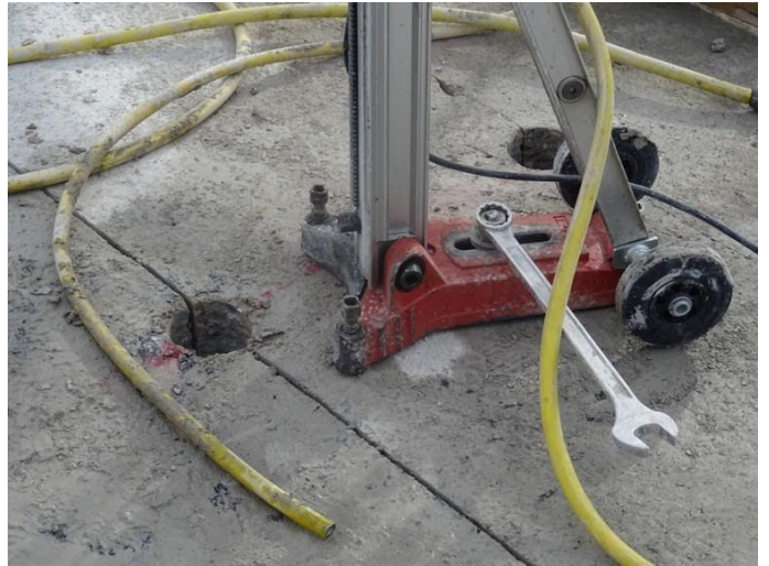
Figure 8. Concrete beam drilling phase.
