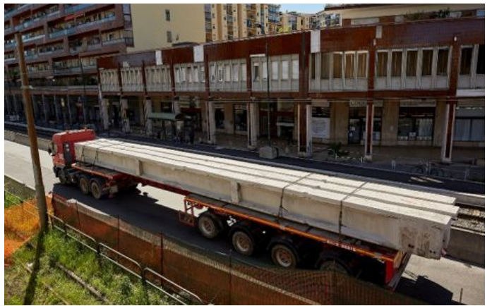
Figure 11. PC beams transportation phase.
