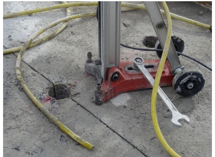
Figure 8. Concrete beam drilling phase.
