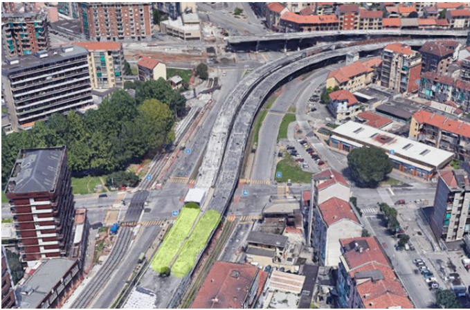
Figure 3. Corso Grosseto viaduct (Turin). The highlighted portion will be tested within BRIDGE|50 research project.
