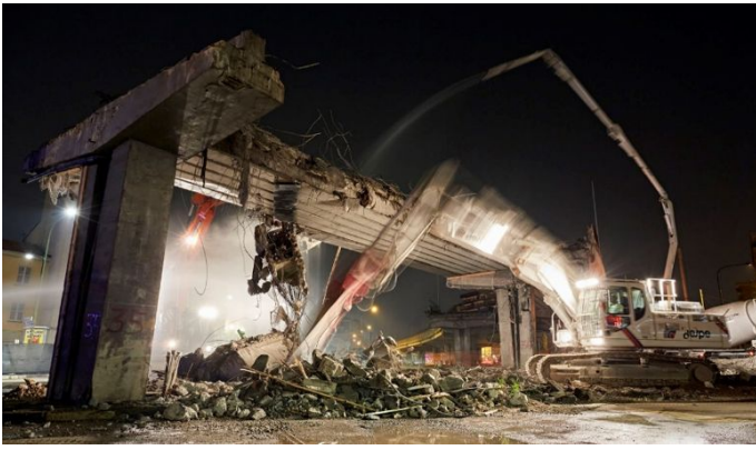
Figure 5. Demolition bridge process using hydraulic pliers.
