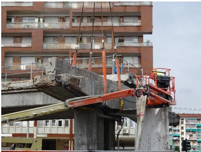
Figure 10. Dismantling phase of pier caps.
