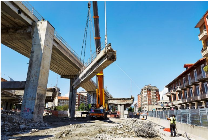
Figure 6. Deconstruction bridge process.
