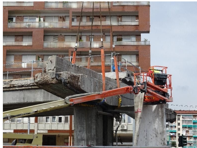
Figure 10. Dismantling phase of pier caps.
