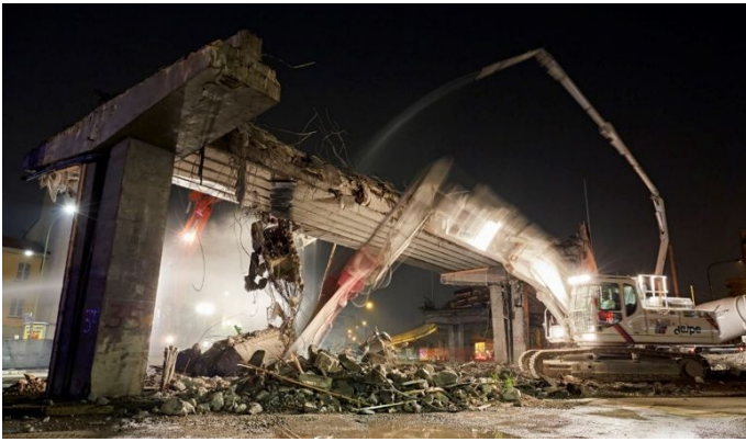
Figure 5. Demolition bridge process using hydraulic pliers.
