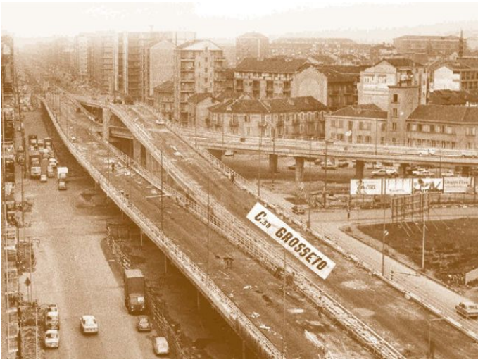
Figure 1. Corso Grosseto viaduct during construction (1970).
