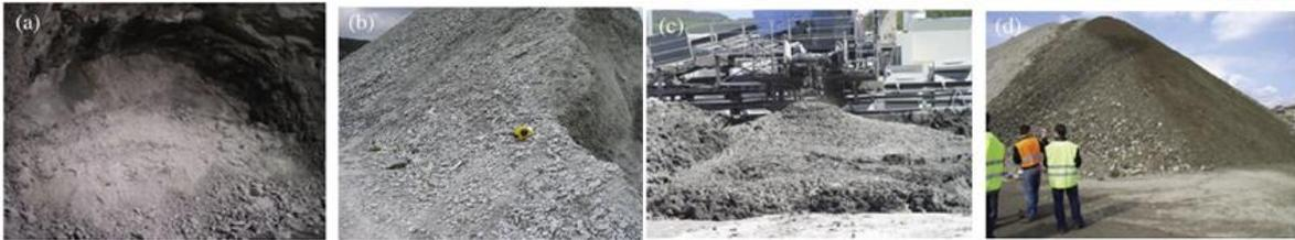
**Figure 1.** Four types of muck suitable for reuse: a) after Drill and Blast in granitic rock mass; b) dump of granitic chips after full face TBM excavation in granitic rock mass; c) EPBS machine excavation in hard soil – soft rock formation, with conditioning; d) dump of coarse soils after mechanized excavation in alluvium.
