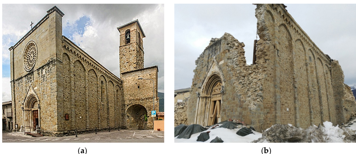
Figure 1. St. Agostino church in Amatrice before (a) and after (b) the seismic earthquake swarm of 2016 in Central Italy.
