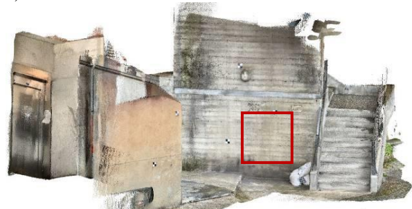
Figure 8. Portion of the wall where roughness and density are computed on an area of 1 m 2 .
