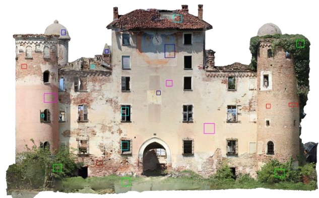
Figure 9. Training areas selected by the user through the user interface. Legend: magenta=plaster, navy=fresco, red=brick, brown=brick with lacks, blue=stone, lime=vegetation, cyan=other.
