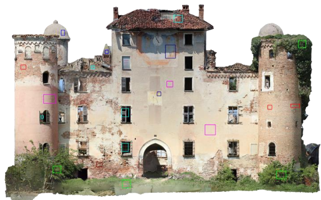
Figure 9. Training areas selected by the user through the user interface. Legend: magenta=plaster, navy=fresco, red=brick, brown=brick with lacks, blue=stone, lime=vegetation, cyan=other.
