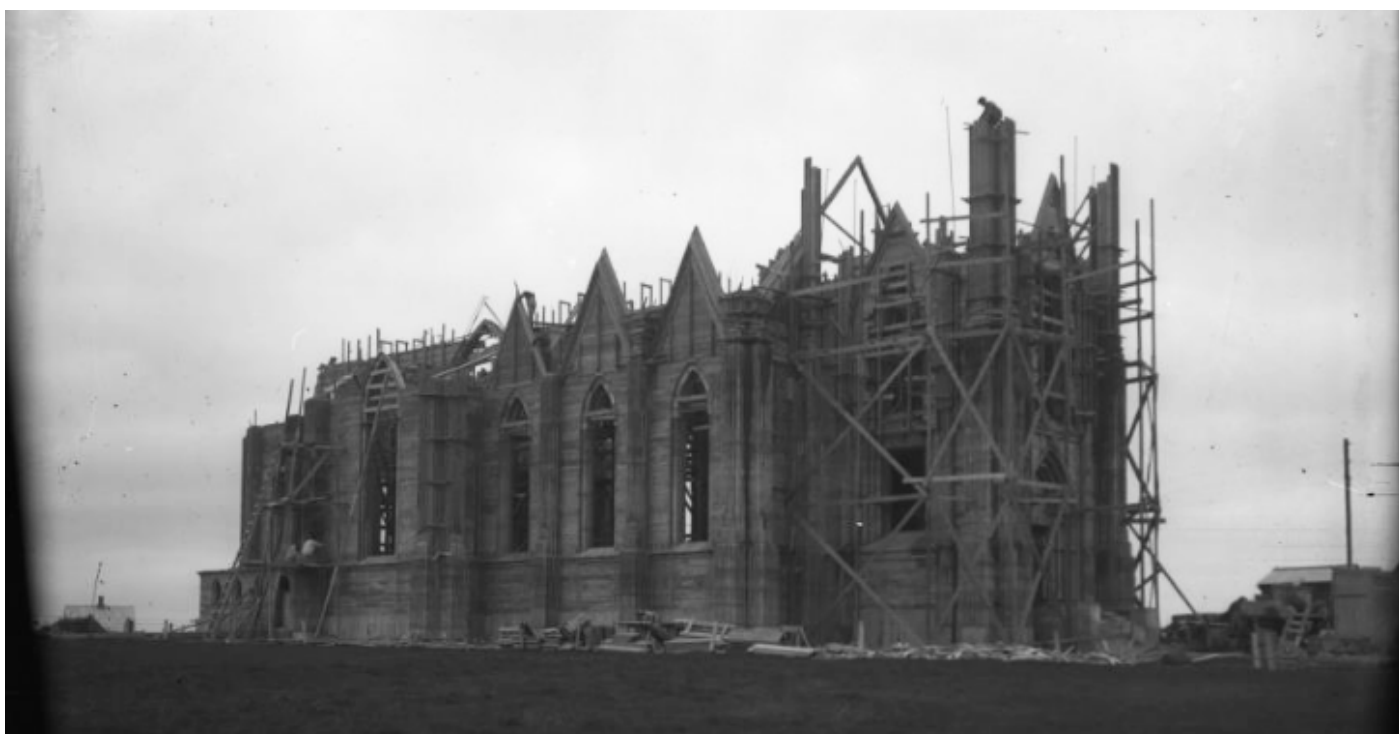
Fig. 21a–21b – The church in construction, 1927–28. Þjóðminjasafn Íslands/National Museum of Iceland.
