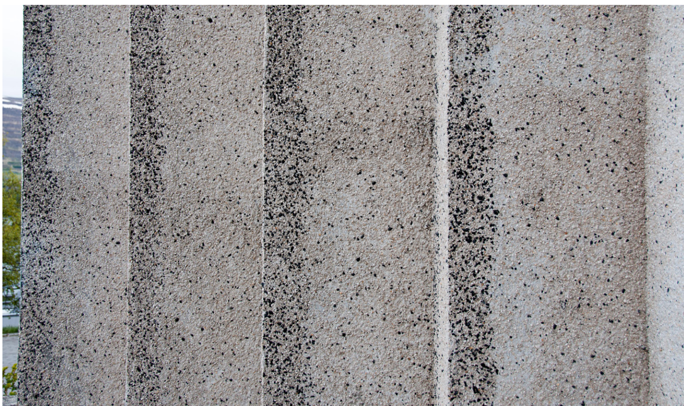
Figg. 40a–40b – Steining render of the church of Akureyri. Details of the obsidian splinters in contrast with quartz fragments. Photos by Sofia Nannini, 2019.
