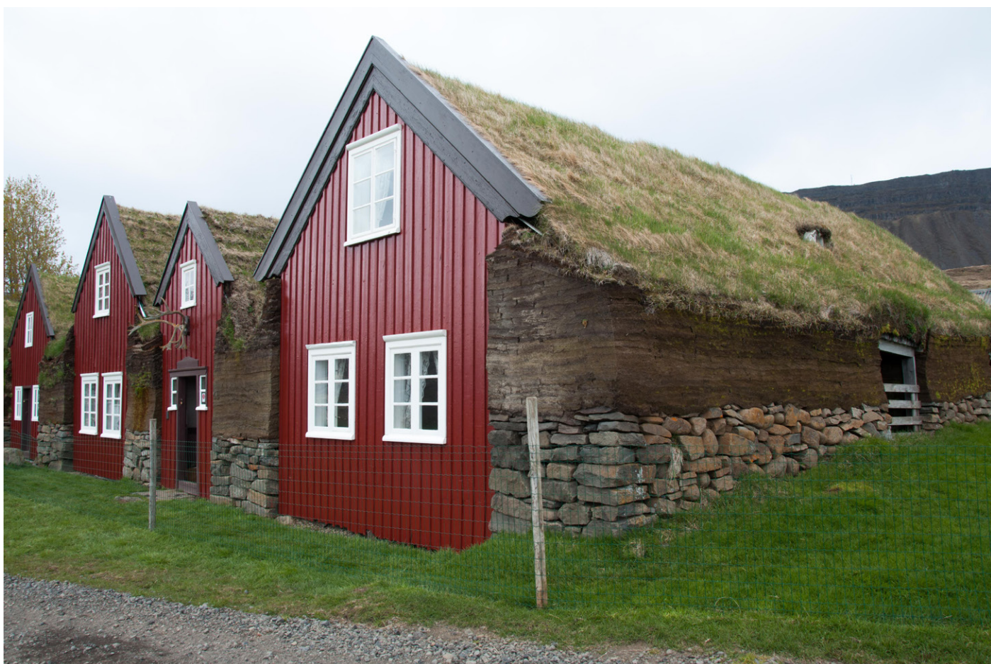
Fig. 4a–4b – “Gabled house” or burstabær in Bustarféll, Vopnafjörður. Originally built in the late eighteenth century, it was inhabited until 1966. Now it is preserved by the National Museum of Iceland. Photos by Sofia Nannini, 2019.
