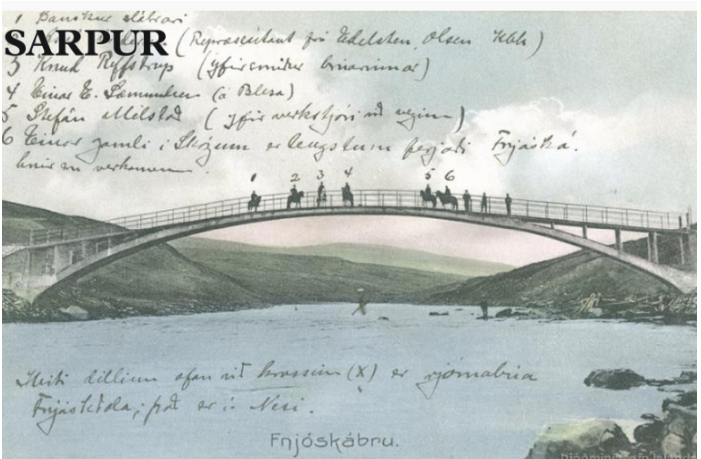
Fig. 37 – Group photo of the workers after the bridge was completed. The man marked with the number 3 is Knud Reffstrup, director of the works. 1908. Þjóðminjasafn Íslands/National Museum of Iceland.
