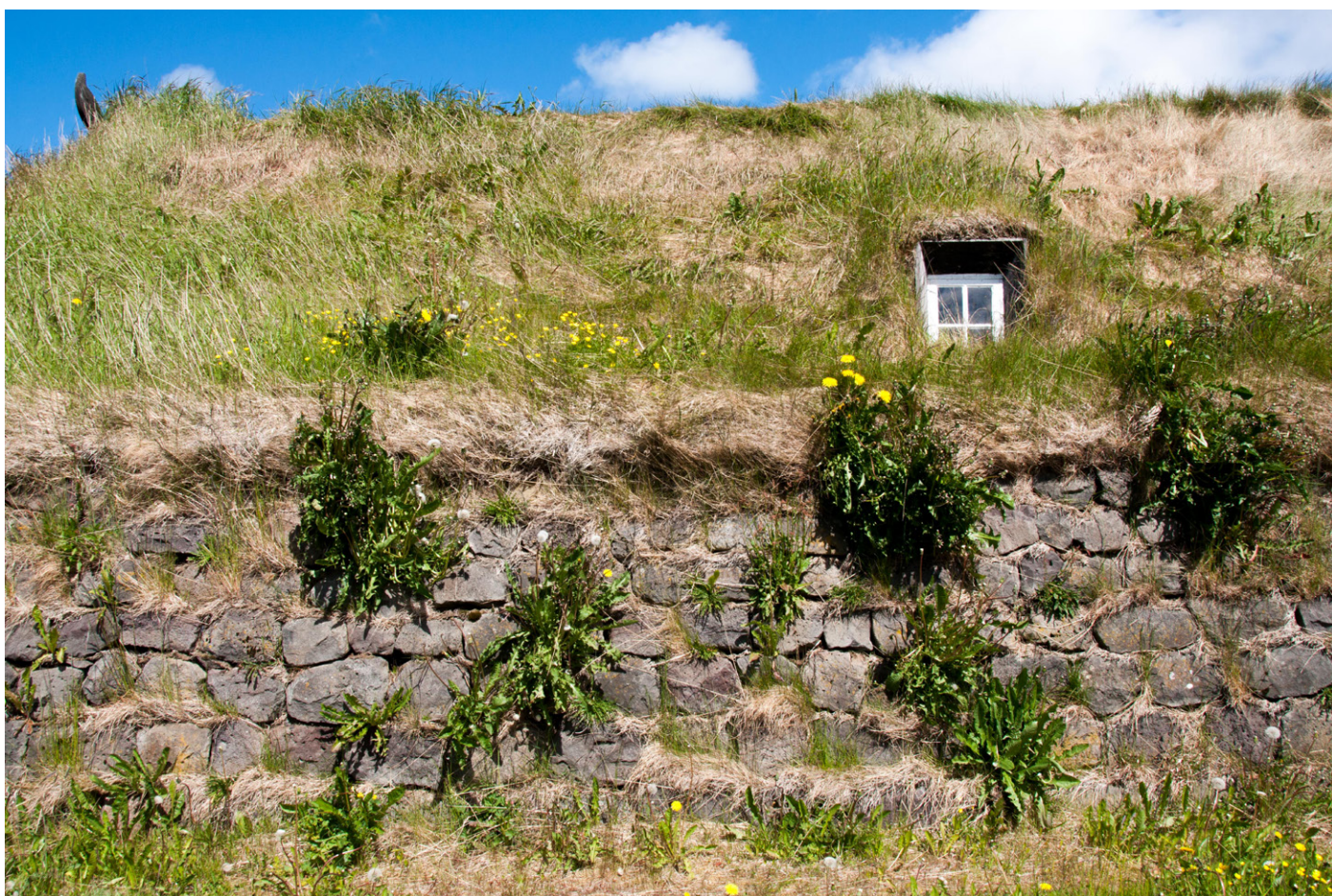
Fig. 1d – Reconstruction of a turf church at the Árbær Museum, Reykjavík. Photo by Sofia Nannini, 2019.
