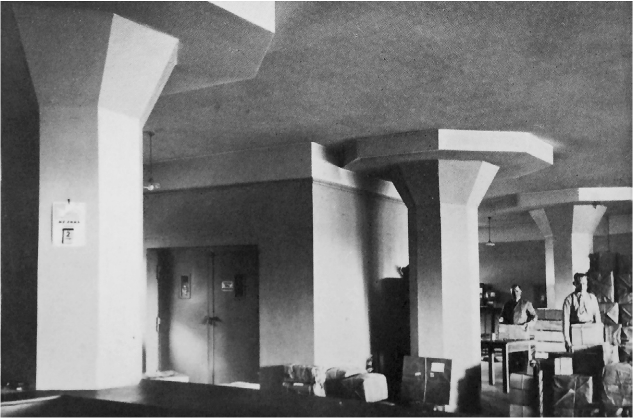
Fig. 4b – Concrete pillars of the warehouse. Sigurður Guðmundsson, “Three New Concrete Buildings in Iceland,” 102.
