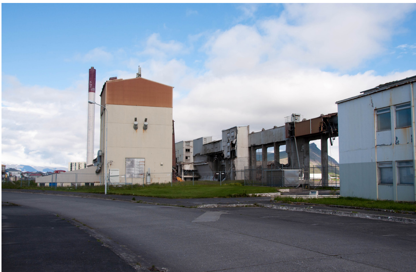
Fig. 52a – The State Cement Works in Akranes before its demolition. Photo by Sofia Nannini, 2018.
