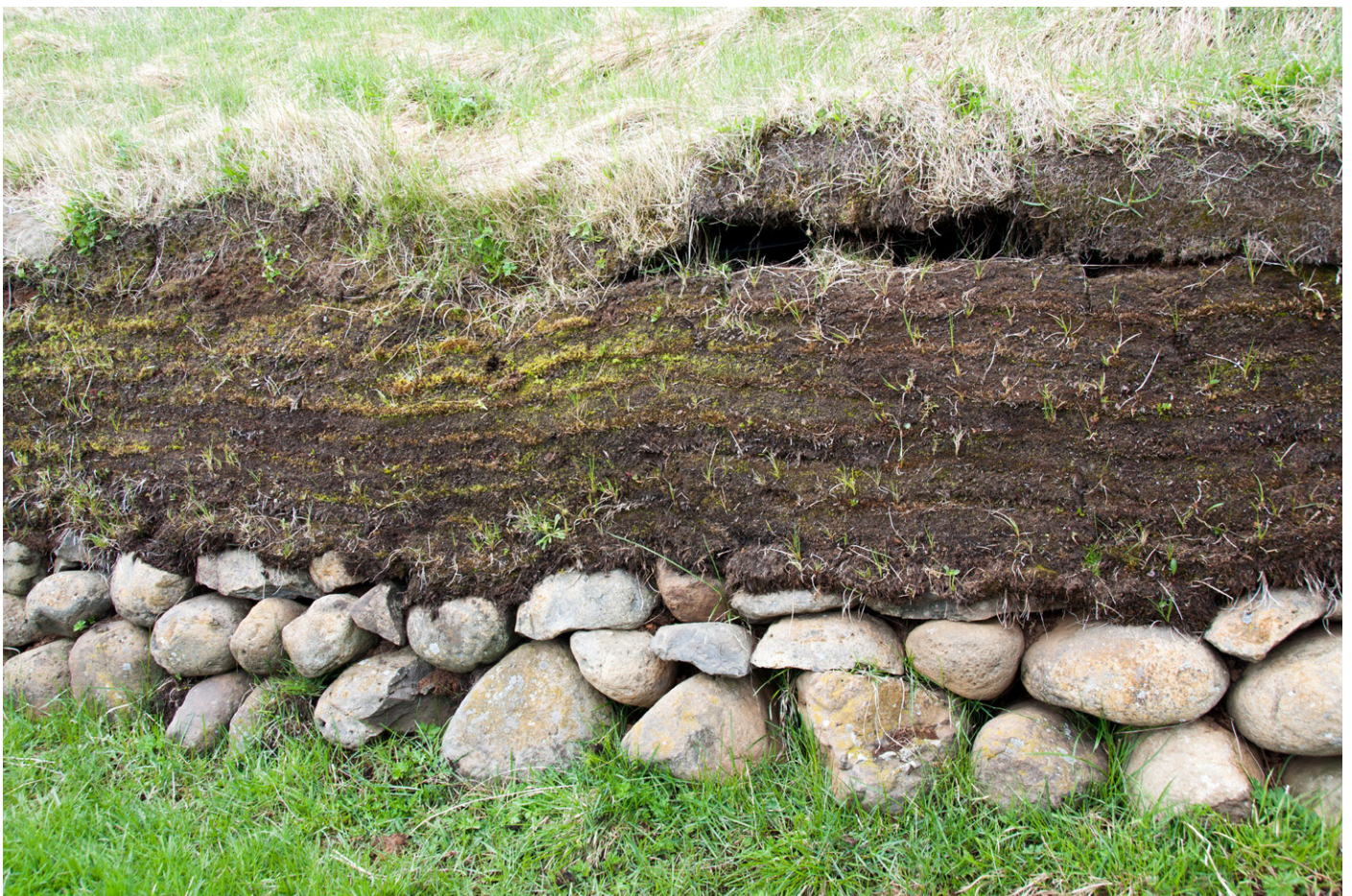
Fig. 2b – Detail of an outer turf wall, Bustarfell, Vopnafjörður. Photo by Sofia Nannini, 2019.
