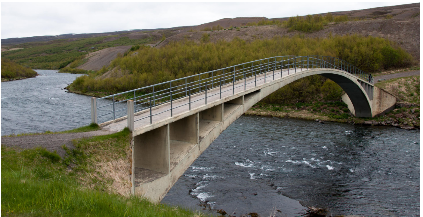
Fig. 38 – The bridge over the Frjóská river. Photo by Sofia Nannini, 2019.
