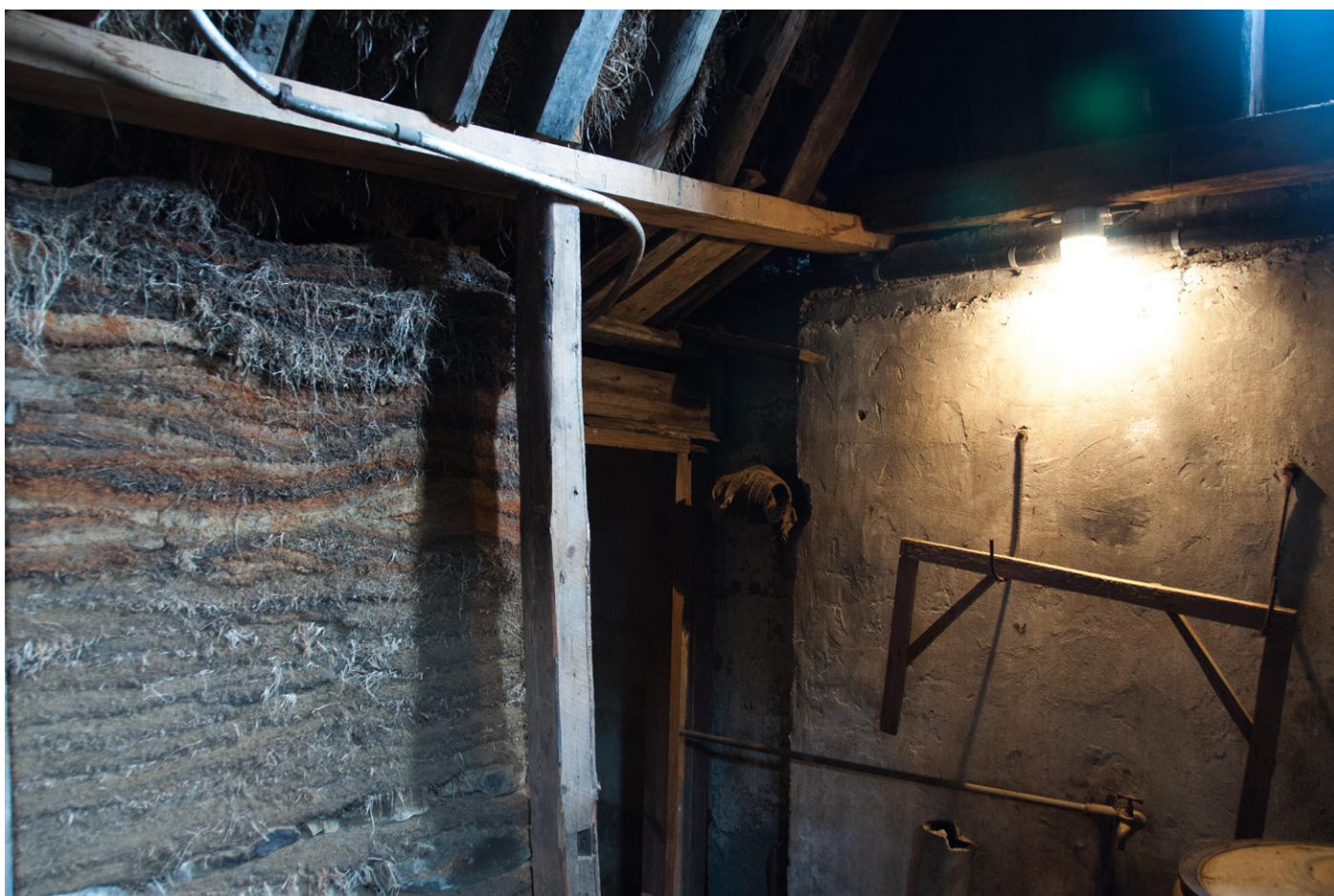
Fig. 13 – Farmhouse (now museum) at Bustarféll, Vopnafjörður. The turf and concrete walls in the former kitchen and laundry room. Photo by Sofia Nannini, 2019.
