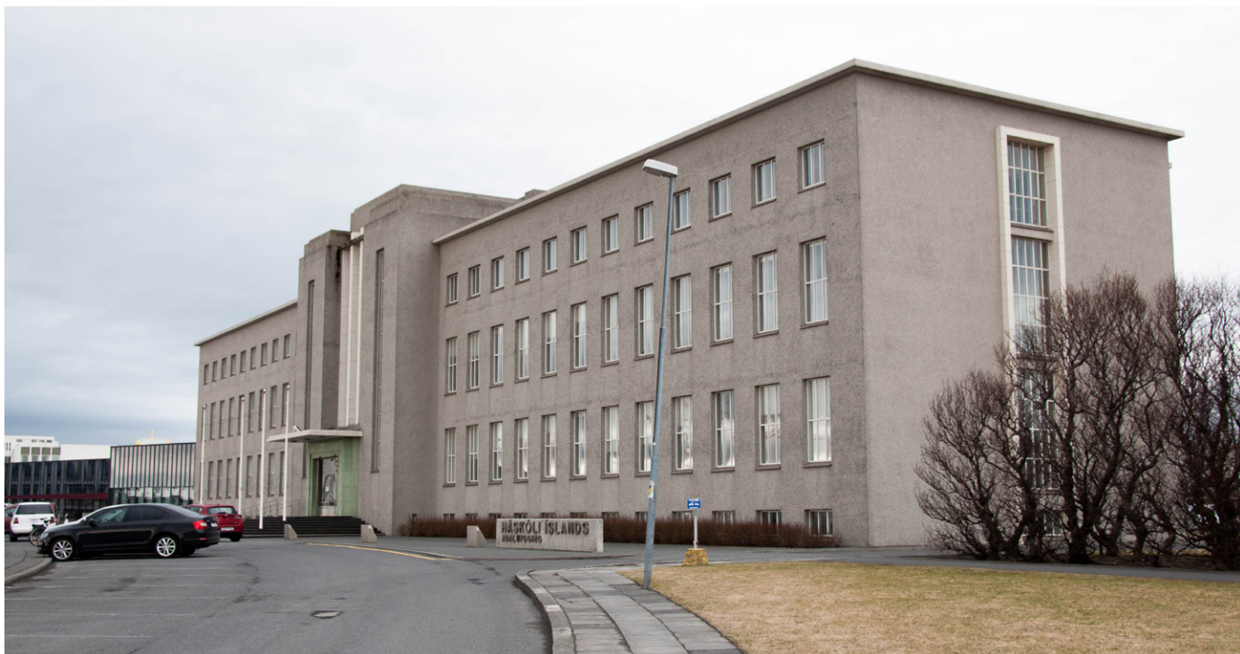
Fig. 42c – The main building of the University of Iceland, 1934–40. Photo by Sofia Nannini, 2018.
