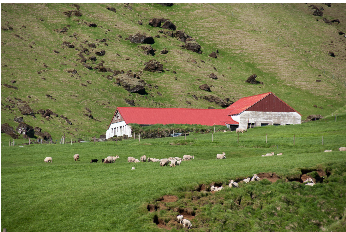
Fig. 16g – Concrete farm with side turf wall at Skógar, South Iceland. Photo by Sofia Nannini, 2019.
