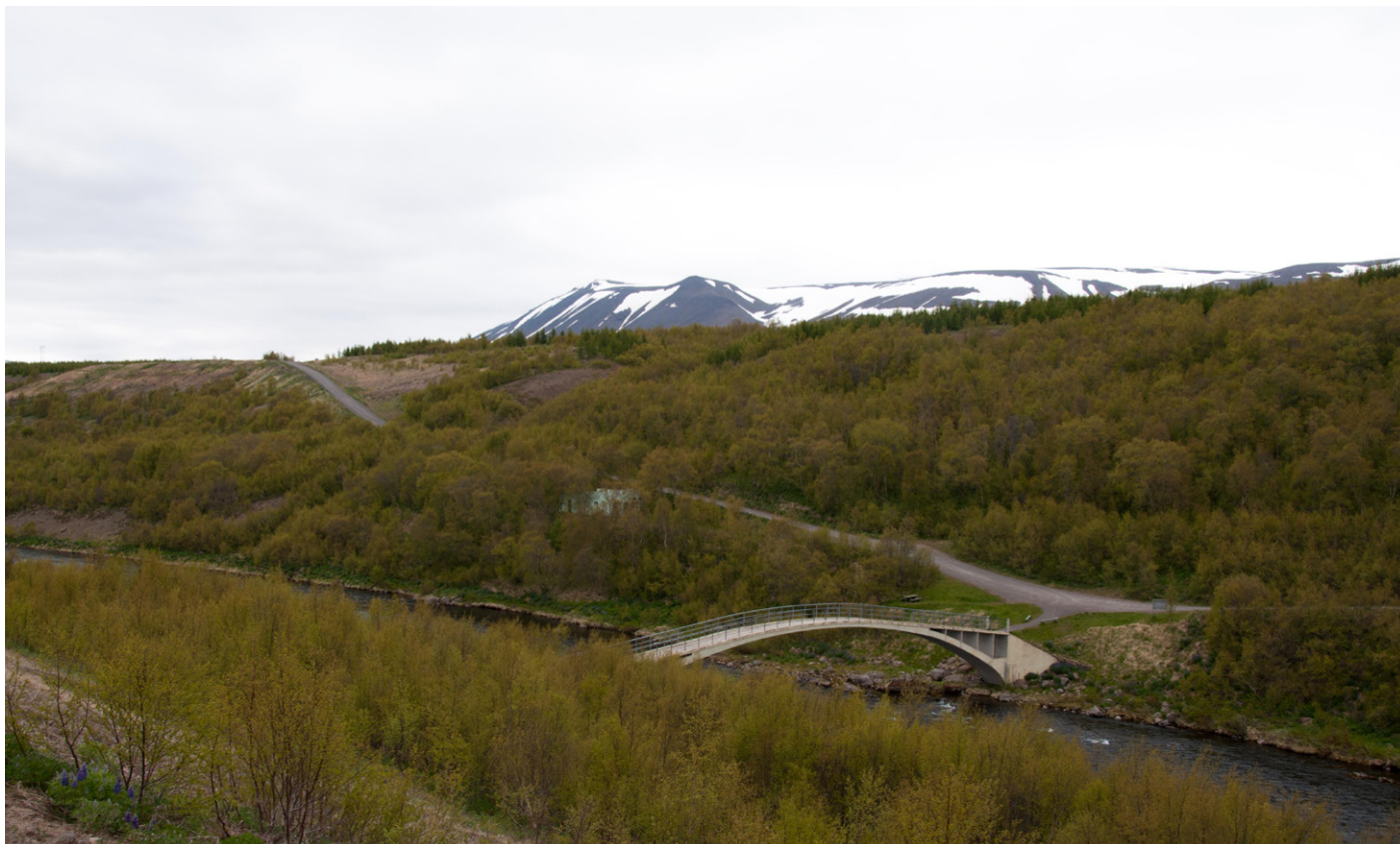
Fig. 34a – Bridge over the Fnjóská river, photo by Sofia Nannini, 2019. The bridge was restored in 1993.
