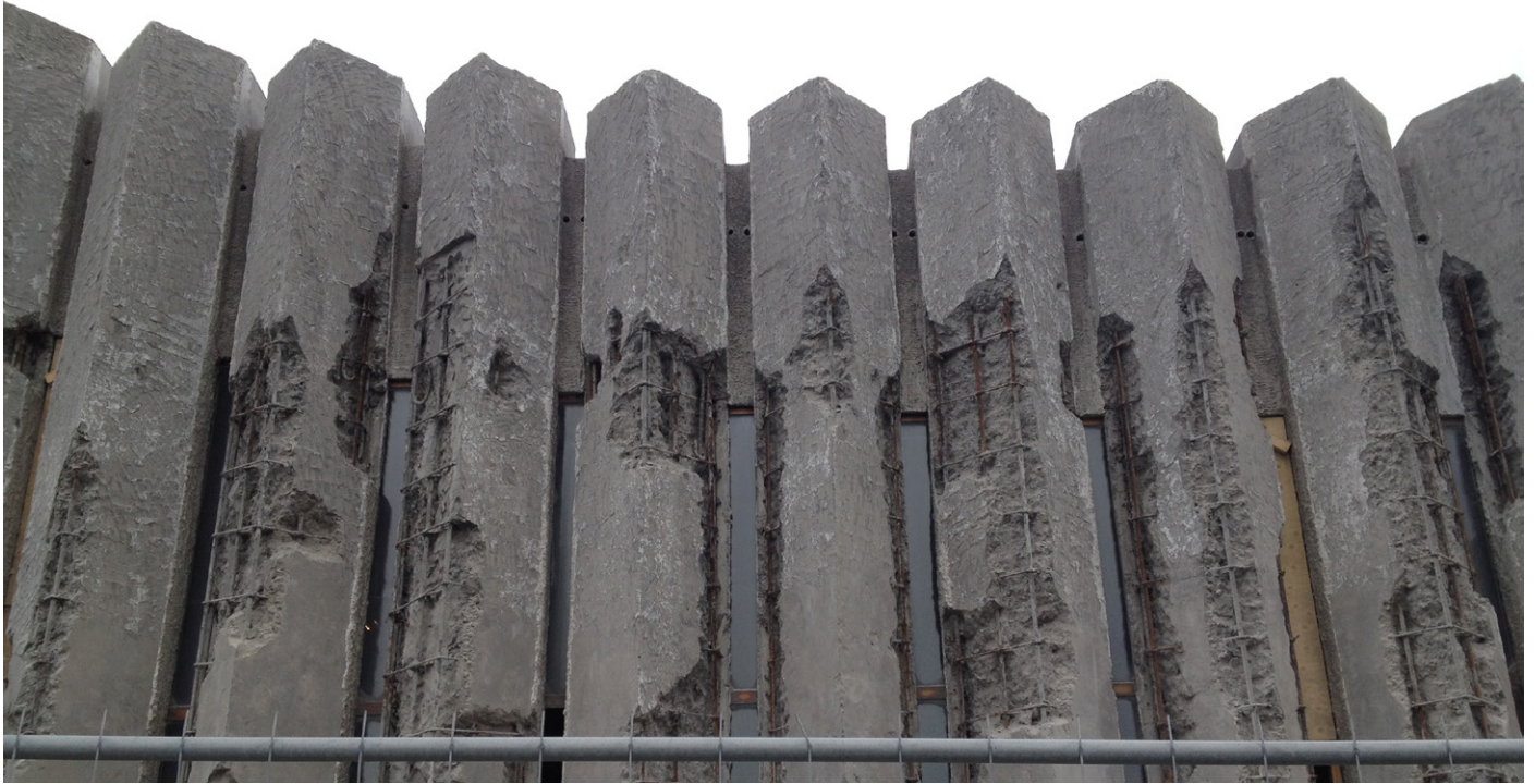
Fig. 12 – Renovation works on the church of Hallgrímur, Reykjavík. Photo by Sofia Nannini, 2016.
