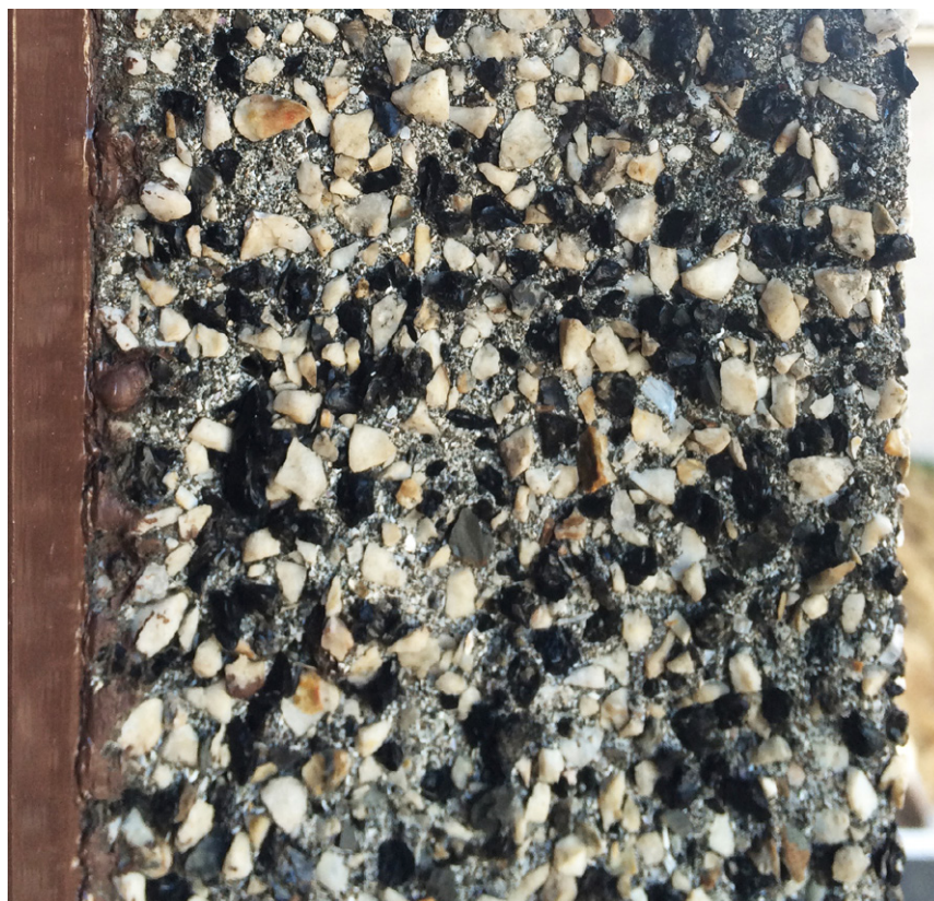
Fig. 41b – Detail of the steining render with fragments of Iceland spar. Photo by Sofia Nannini, 2019.
