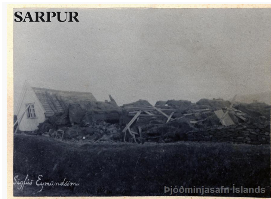
Fig. 1–2–3 – Turf farms destroyed after the earthquakes in Southern Iceland, 1896. Þjóðminjasafn Íslands/National Museum of Iceland.
