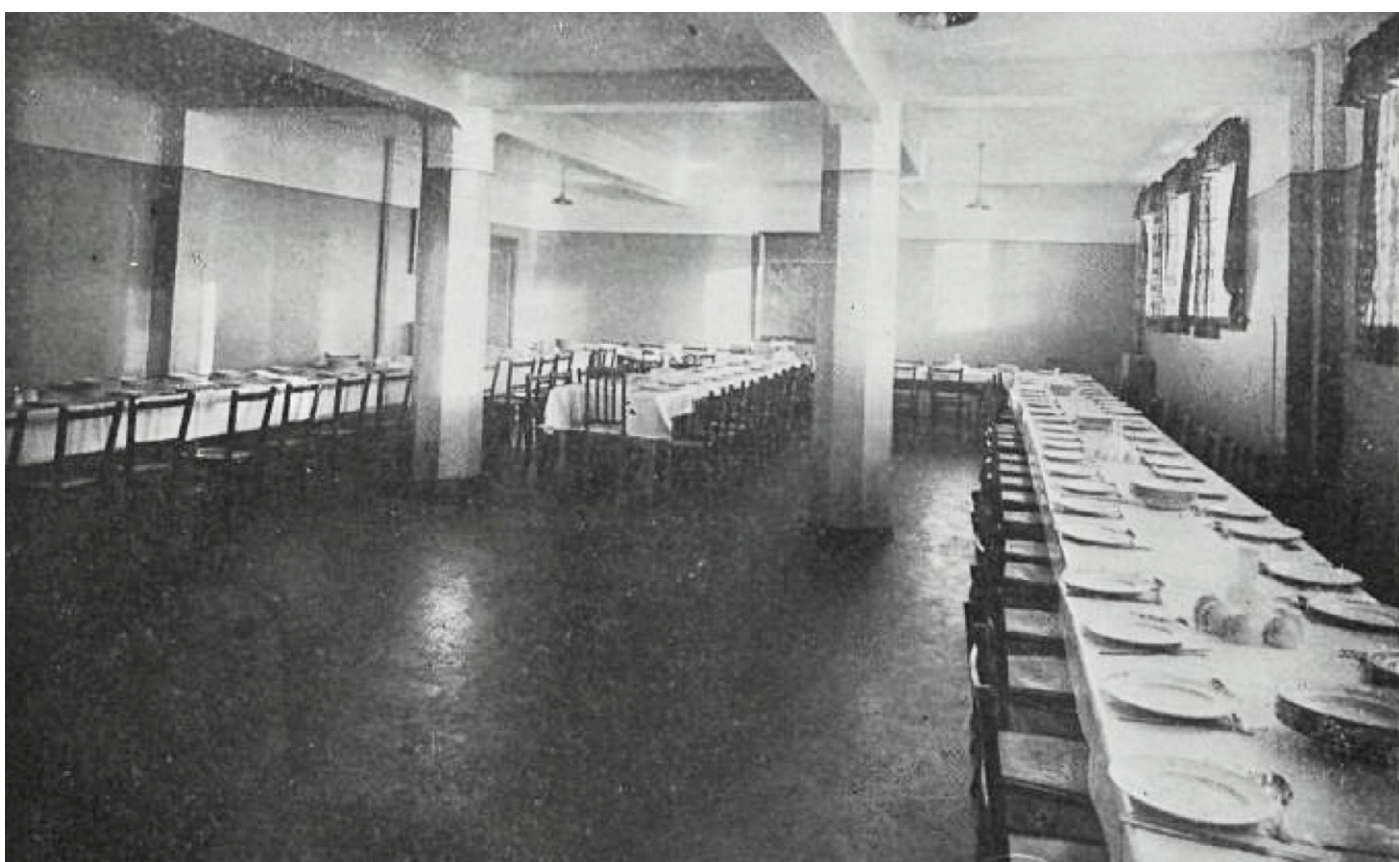
Fig. 13b – Guðjón Samúelsson, School in Laugarvatn, 1929–32. Detail of the inside frame structure. Guðjón Samúelsson, “Íslenzk bygginarlist,” Tímarit Verkfræðingafélags Íslands 18, no. 6 (December 1933): 67.
