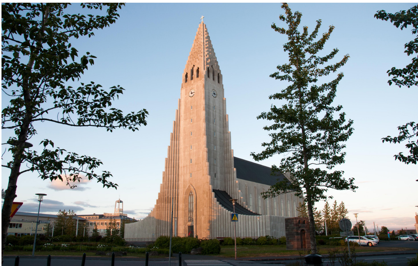
Fig. 23b – Guðjón Samúelsson, Church of Hallgrímur [Hallgrímskirkja], Reykjavík. 1937–86. Photo by Sofia Namini, 2019.
