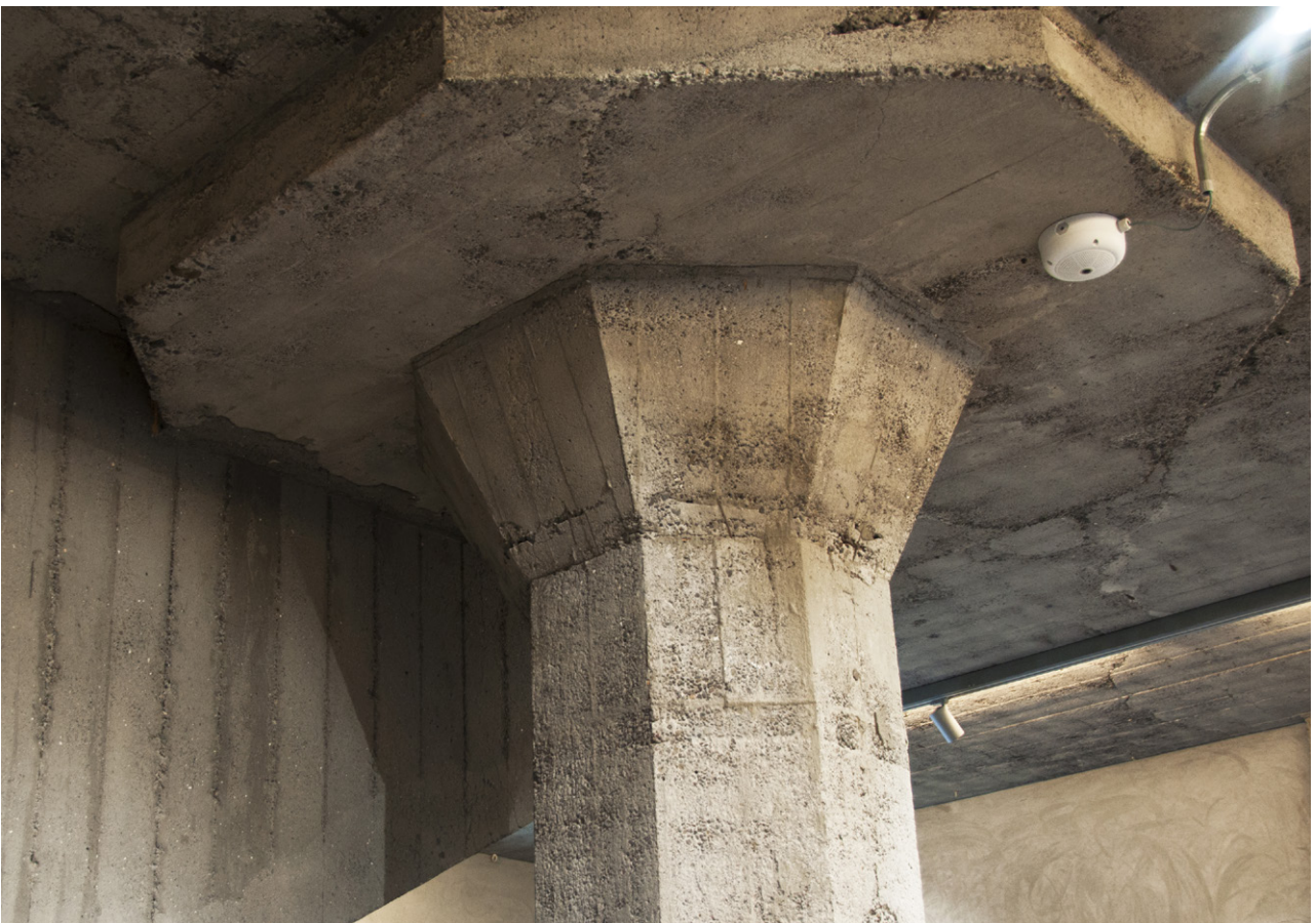
Fig. 4c – The concrete pillars today. The material is damaged and one can often see the presence of very coarse aggregates within the concrete mix. Photo by Sofia Nannini, 2019.
