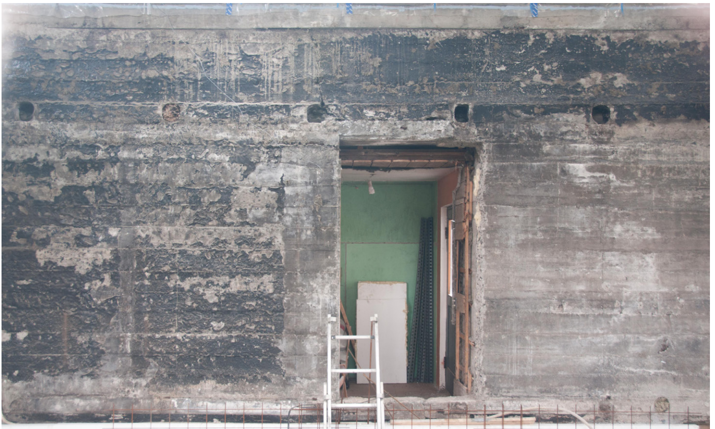
Fig. 22 – Detail of the cast concrete inside the farm. Photo by Sofia Nannini, 2019.
