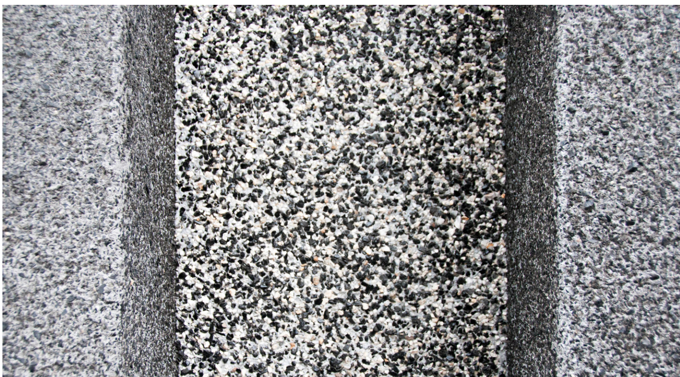
Fig. 38a–38b. Steining render on the National Theatre. The darker shades are related to the presence of obsidian fragments. Photos by Sofia Nannini, 2018.
