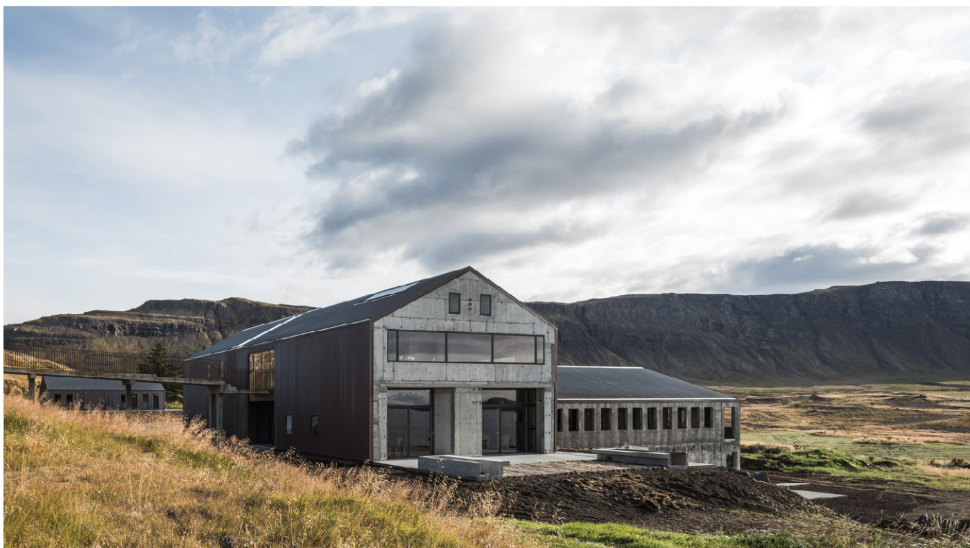
Fig. 11 – Studio Granda, Drangar Renovation (2019). Archdaily , https://www.archdaily.com/925031/drangar-renovation-studio-granda?ad_medium=office_landing&ad_name=article , last accessed 15/11/2020.
