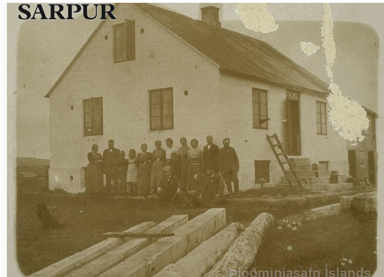
Fig. 17 – Farmhouse made with concrete cast stones, possibly produced by Steinar , ca. 1905–15. Þjóðminjasafn Íslands/National Museum of Iceland.
