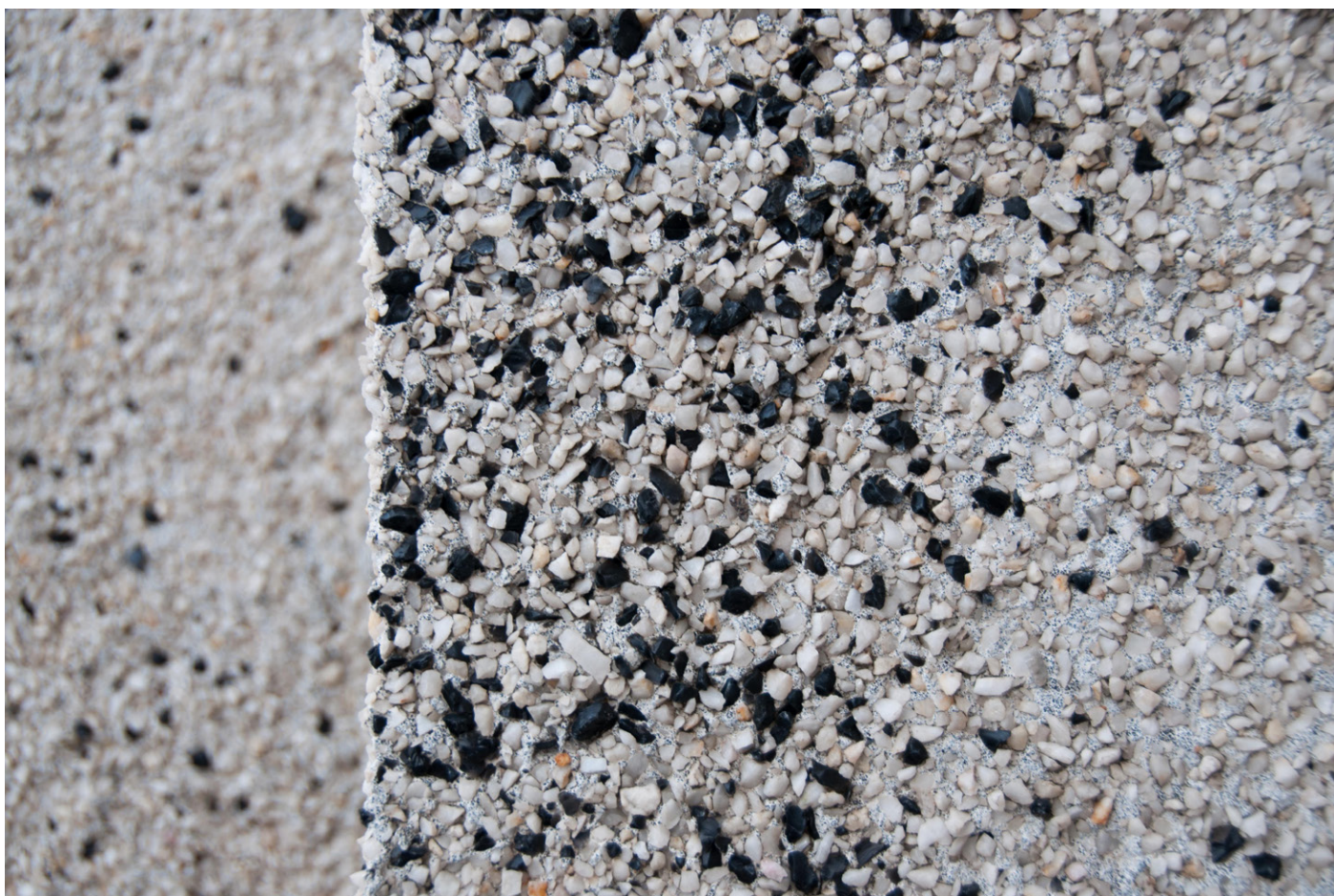
Fig. 40c – Steining render of the church of Akureyri. Details of the obsidian splinters in contrast with quartz fragments. Photos by Sofia Nannini, 2019.
