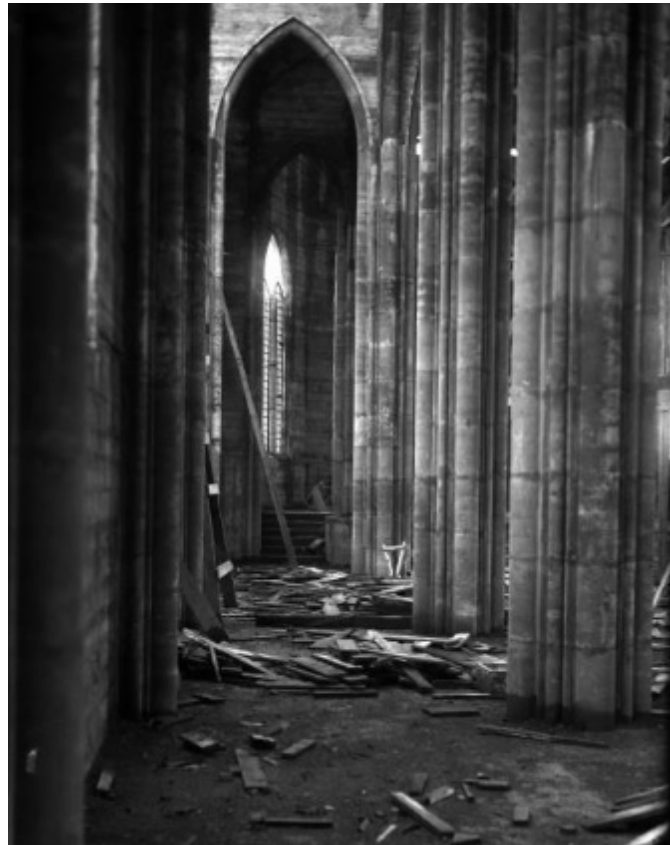
Fig. 20b – The pillars after the construction. In the photo the pillars had not been plastered yet, so the precast blocks are still visible. 1928. Þjóðminjasafn Íslands/National Museum of Iceland.
