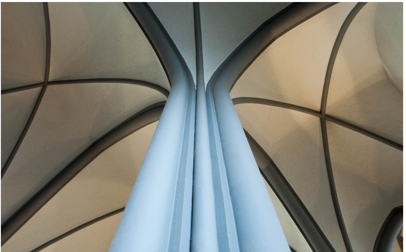
Fig. 20c – The pillars and the vaults today. Photo by Sofia Nannini, 2018.
