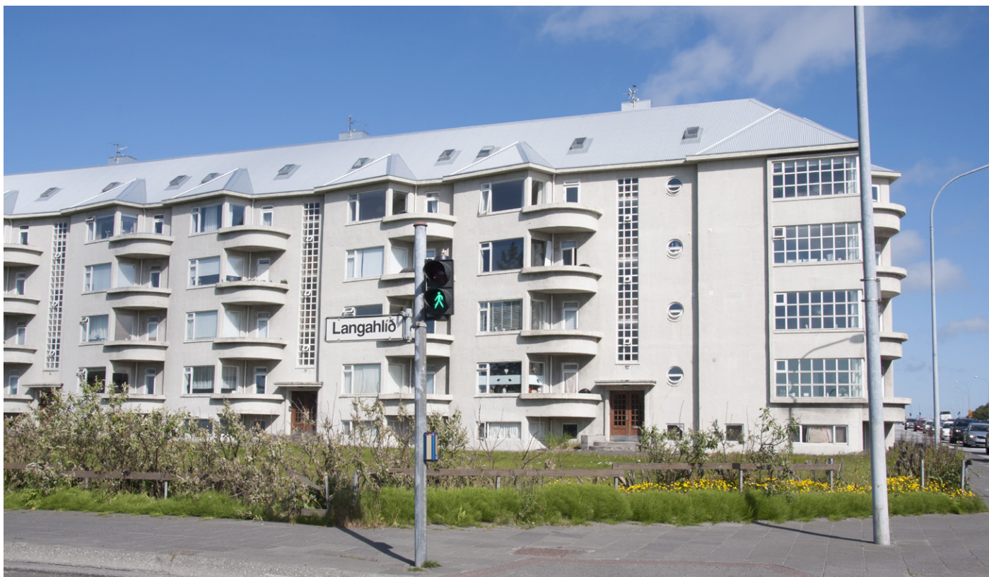
Fig. 47c – Einar Sveinsson and Ágúst Pálsson, Apartment buildings in Miklabraut/Langahlíð 19–25, Reykjavík, 1945–49. Photo by Sofia Nannini, 2019.
