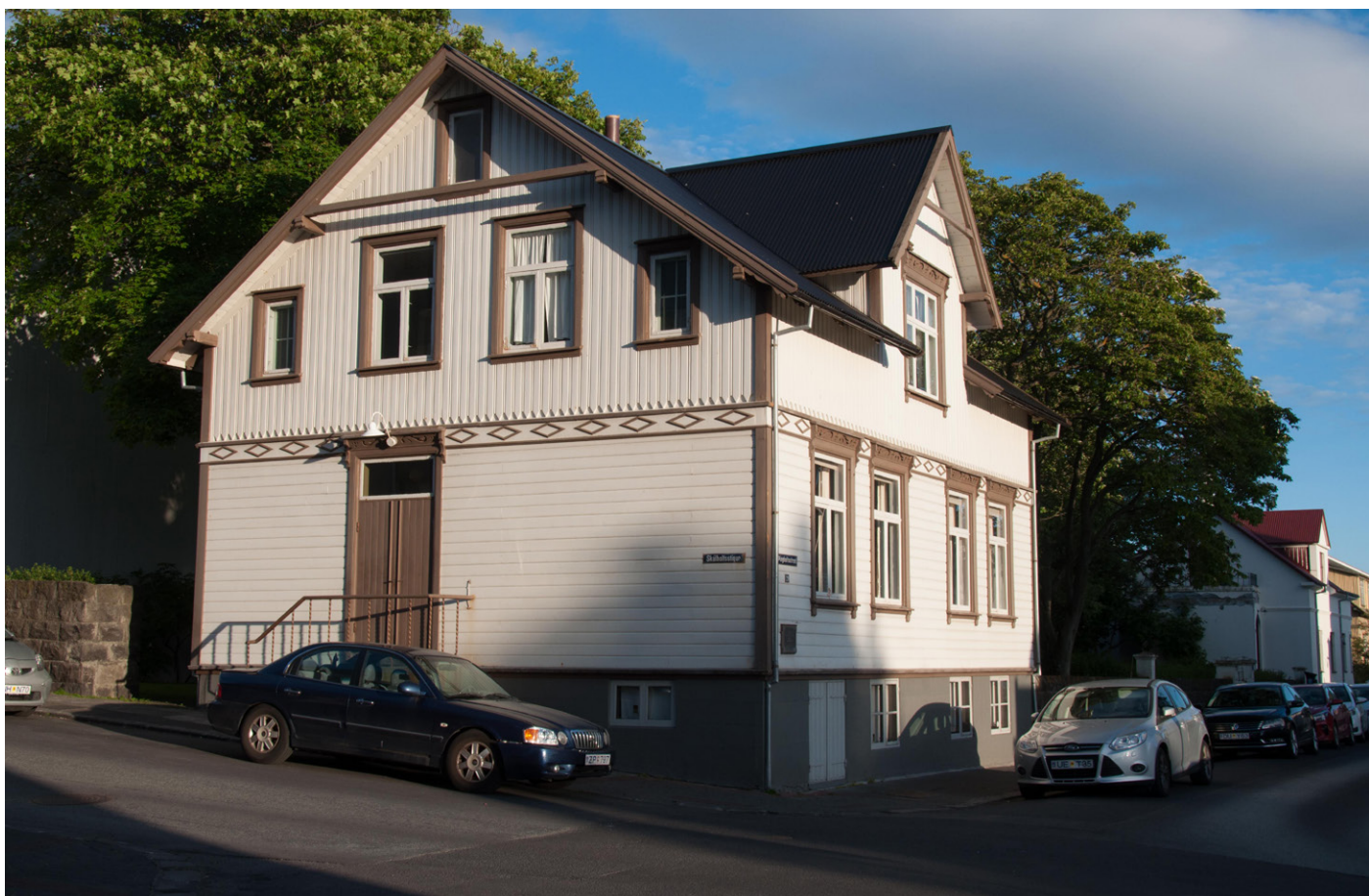
Fig. 5b – House in Þingholtsstræti 29, Reykjavík, “catalogue house” prefabricated in Norway and built in 1899. Photo by Sofia Nannini, 2019.
