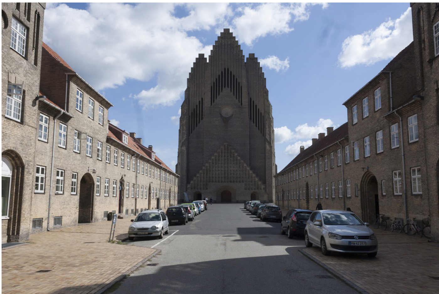
Fig. 26 – P. V. Jensen-Klint, Grundtvig Church, Copenhagen, 1921–40. Photo by Michele Barale, 2018.
