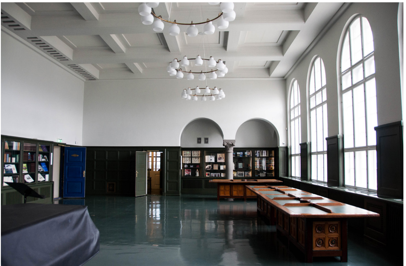
Fig. 57 – The reading room covered by a coffered reinforced concrete slab. Photo by Sofia Nannini, 2018.
