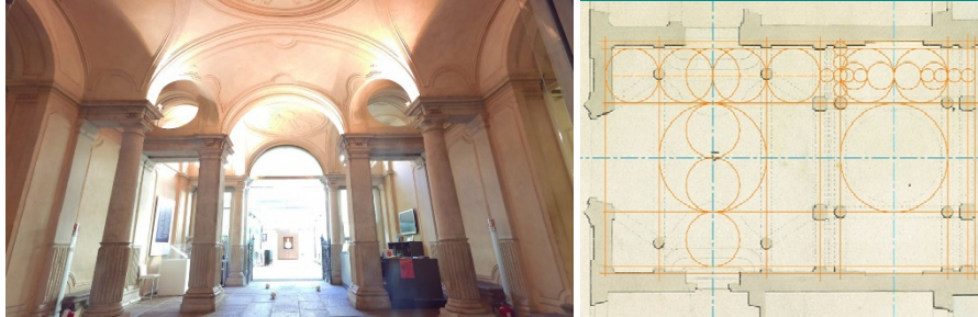
Fig. 1. Atrium of Palazzo Mazzonis in Turin; excerpt of the survey drawing dated 1st July 1845 with superimposition of graphical analysis. Source: Archivio Storico del Comune di Torino, Tipi e dis., cart. 63, fasc. 9, dis. 1, tav III. Photo: F. Natta. Graphic processing: F. Ronco.
