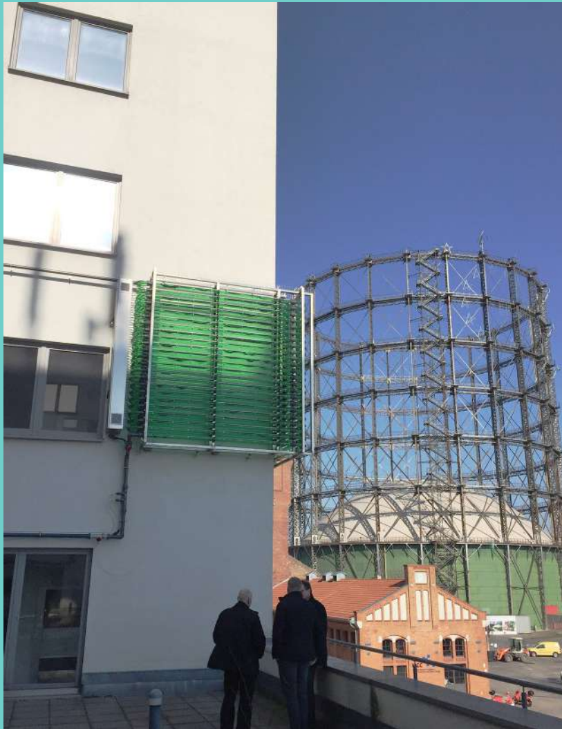
Figure 7.53. Due to its exposition, the photobioreactor can be regulated adaptively with a controller. Retrieved from https://www.gfps.com/content/dam/gfps/master%20Content/Pictures/Company/References/MINT_02.jpg
