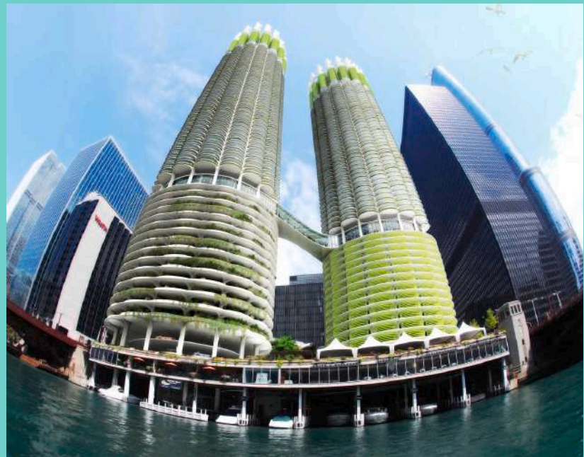
Figure 7.89. Fisheye render view of the retrofitted Marina City's Towers. Adapted from Archdaily website, 2011, retrieved from https://www.archdaily.com/191229/algae-green-loop-influx-studio/01-fisheye Copyright 2011 by Influx Studio.
