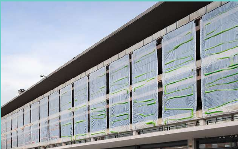
Figure 7.78. The curtain is composed of several bioplastic modules, each of them digitally designed.
