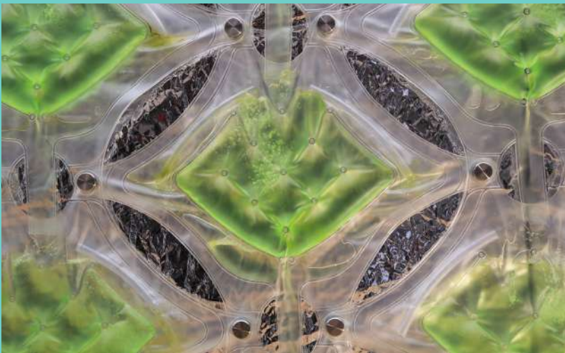
Figure 7.41. Detail of the modules. Water flows from one module to the other through simple spouts.
