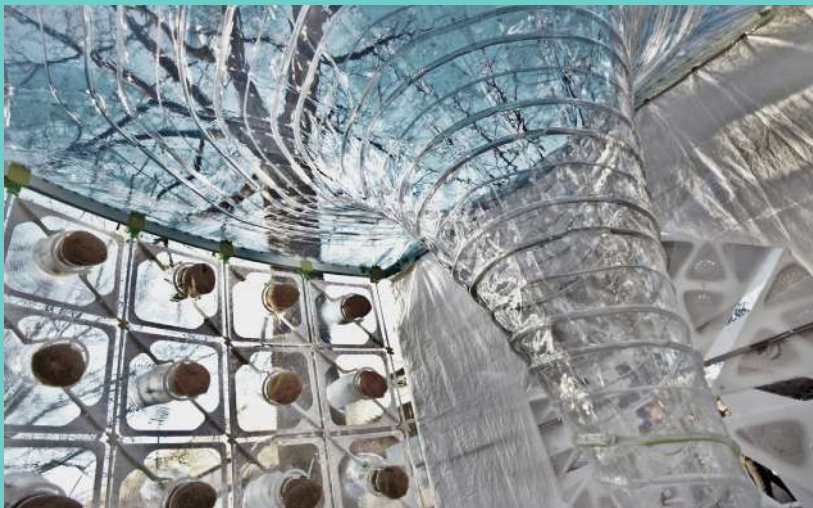
Figure 7.33 (Above). The three separate spirals. 1. Carbon dioxide; 2. Microalgae ascension; 3. Microalgae descension. All the pictures in this page are adapted from inhabitat website, 2016, retrieved from https://inhabitat.com/algaevator-transforms-algae-production-into-a-beautiful-work-of-art-and-architecture/ Copyright 2016 by Iwan Baan.
