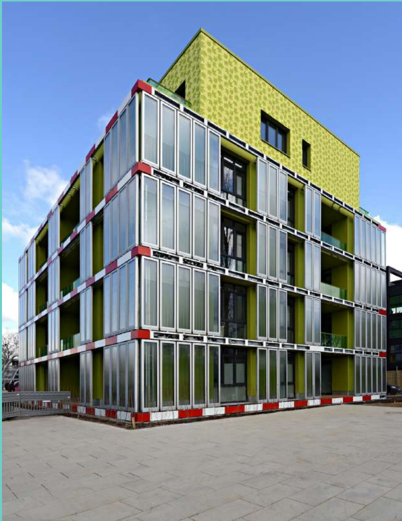
Figure 7.30. The south-west and the south-east sides of the building are characterized by a second layer of photobioreactors (129 in total), that are set into the façade. All the pictures in this page are adapted from Archello website, 2013, retrieved from https://archello.com/project/biq-house/ Copyright 2013 by ARUP.
