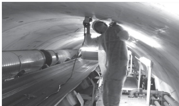
Figure 27 - Georadar test in Roma Metro C construction site (Pelizza et al., 2012).
