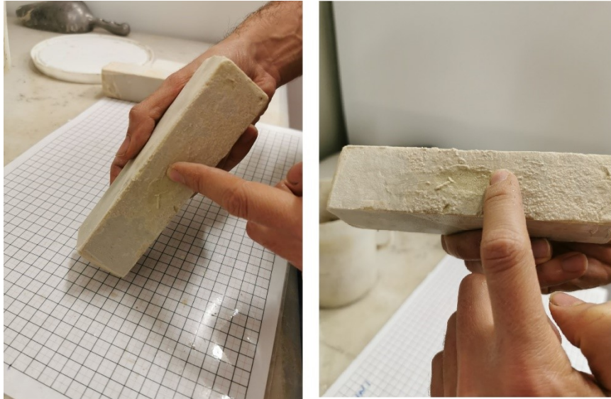
Figure 81 - Deteriorated external layer of the sample.
