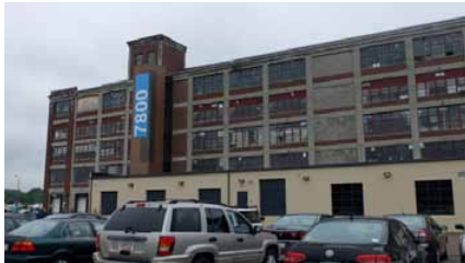
Figure 5. 7800 Susquehanna Street. Pittsburgh. Source: (Ingaramo R. 2018)
