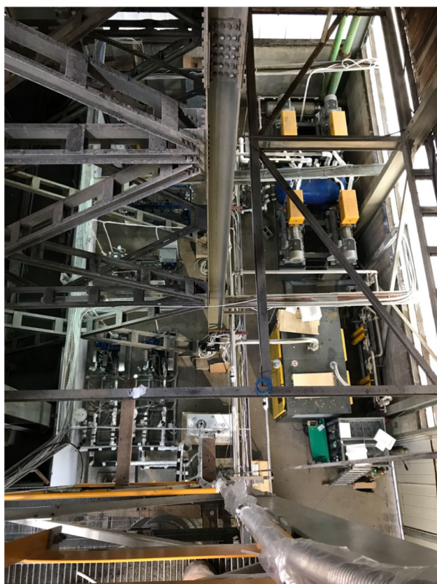
Fig. 11 Aerial view of the prototype Aria plant located in the Laveria building of the Carbosulcis mine, Nuraxi-Figus site. From bottom left, clockwise, the liquid pumps, the cryocoolers, and the gas compressor
