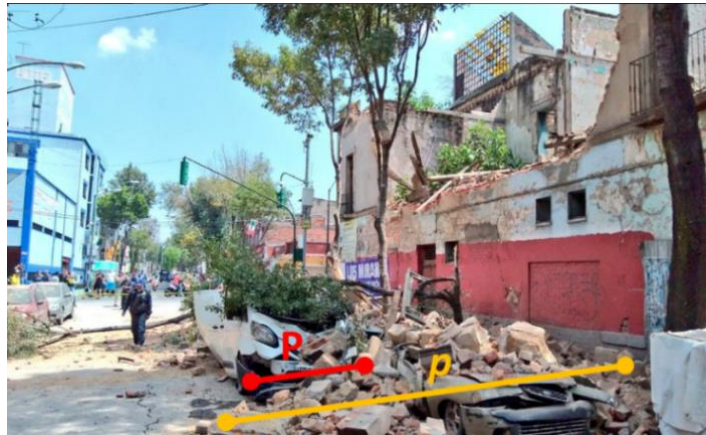
357 Figure 6. Example of debris extension evaluation.
