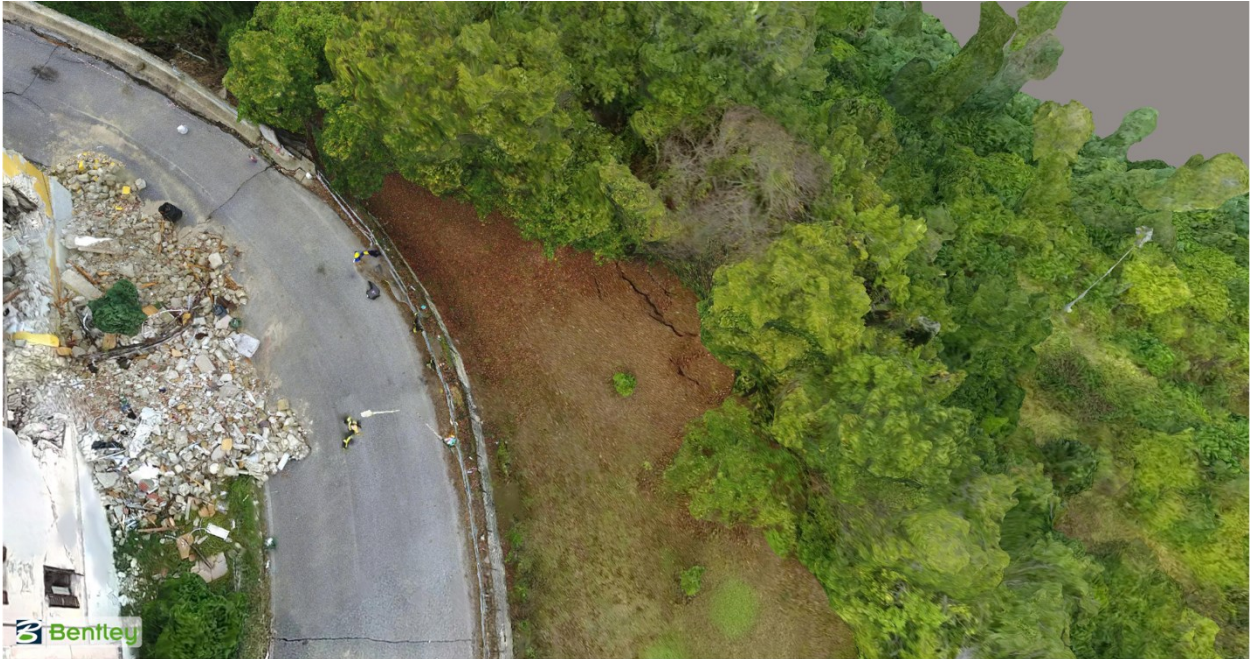
Figure 4.45. Model image of the cracks found in the silty-sandy fillslope located adjacent to the eastern walls of Accumoli. Crack widths range from 5 to 14 cm (42.69406 N 13.25019 E).
