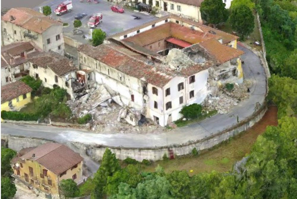
Figure 5.3. Excerpt of the 3D model with the most damaged portion of Accumoli (easternmost part of the village).
