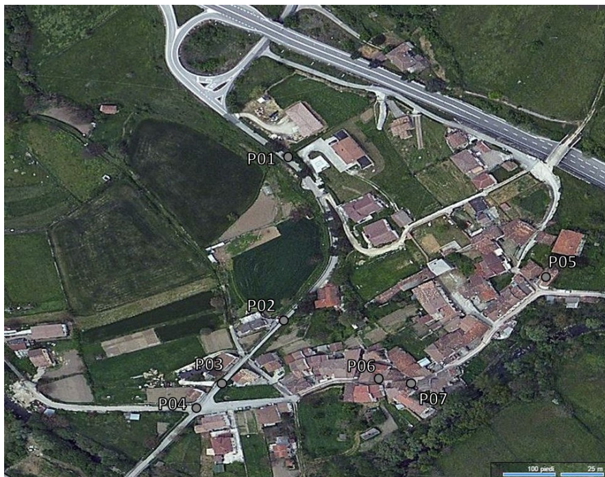
Figure 5.48. Locations of representative structures inspected in the hamlet (see Table 5.11 for details)
