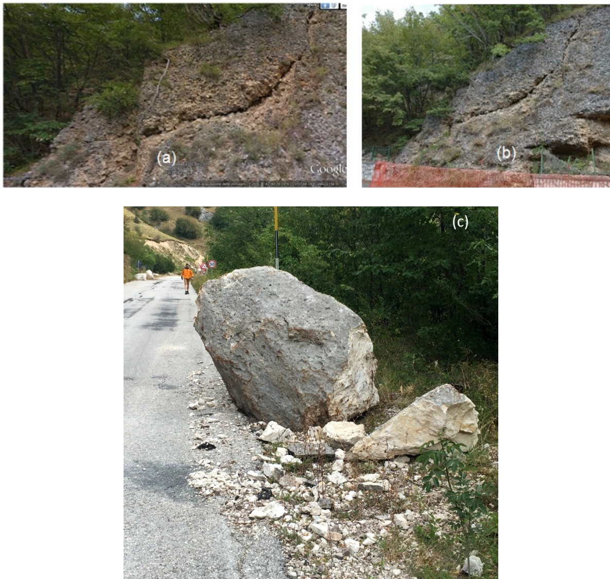
Figure 4.17. Large block of breccia (a) before the earthquake (image courtesy of Google 2016), (b) after the earthquake, and (c) example of rock fall below the Plano Grande on SP477. A large 2-m block of limestone crossed the road came to rest on the downslope side of the roadbed below a prominent outcrop of limestone (42.76729 N 13.16983 E).
