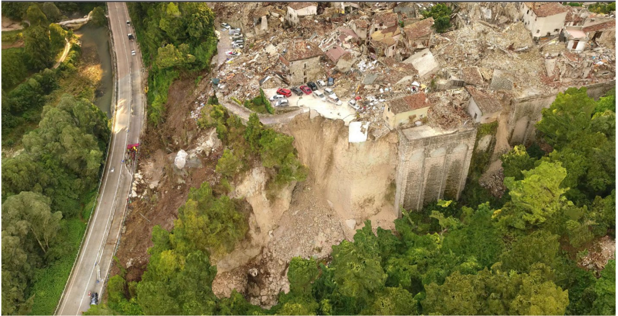
Figure 4.30. 3D model of a slope failure in Pescara del Tronto possibly caused by a retaining wall collapse (42.75109 N 13.27208 E).
