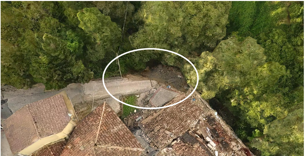
Figure 4.33. Model image of a landslide following a corner retaining wall failure in Pescara del Tronto (42.75166 N 13.27111 E).
