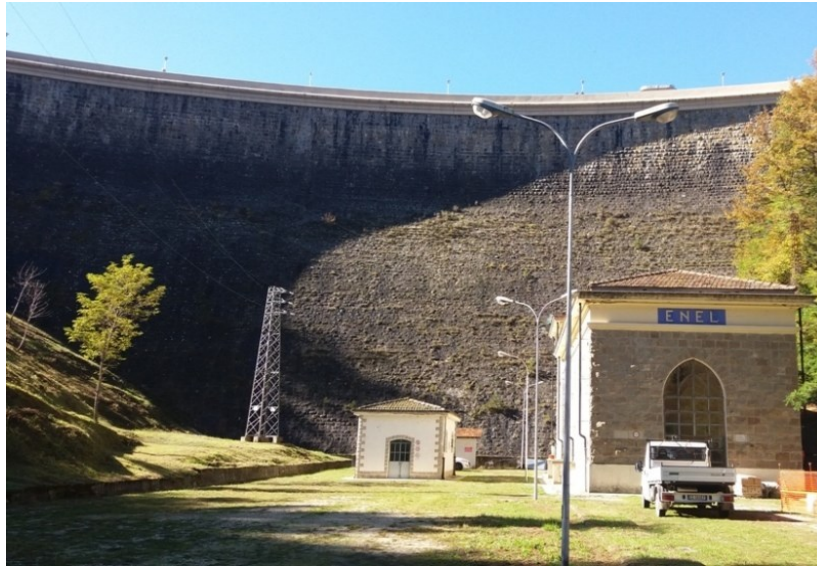
Figure 7.12. Downstream face of Scandarello dam, with the homonymous station for hydroelectric power generation located at the foot of the dam (October 19, 2016).
