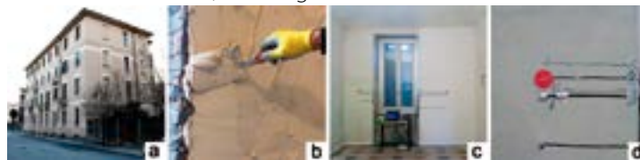
Figure 3 – a) The ATC building selected as pilot site; b) the plaster application; c) the walls selected for the monitoring; d) the sensors adopted for the monitoring
