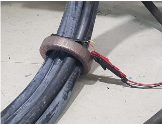
Fig. 5. Test specimen installed on the power converter cables.
