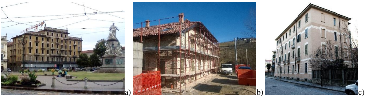
Figure 2. a) Ex Albergo di Virtù case study selected for plaster A (picture from Bianco et al. , 2015); b) the building during the refurbishment and selected for plaster B (picture from Fenoglio et al. , 2018); c) the ATC building selected for the plaster C (picture from Fantucci et al. , 2019).
