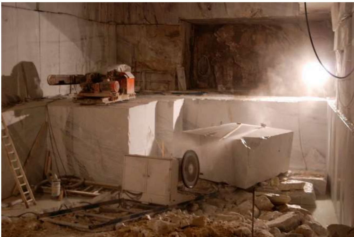
Figure 8. Chain cutting machine (on the top of the bench) operates in an underground extraction site (Lasa quarry), while a diamond wire saw performs a squaring operation.
