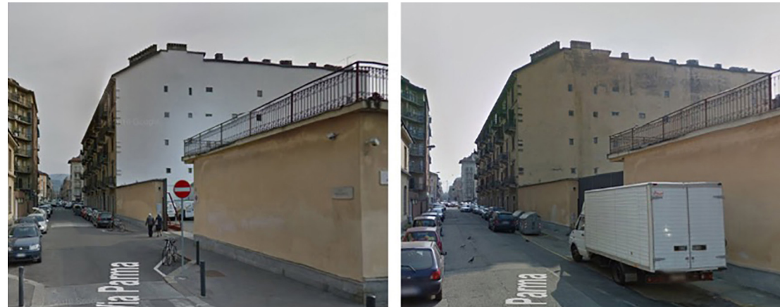
Fig. 14 – TOWard 2030 project, Mantra, Via Parma 24, Turin. Objective 13 Fight against climate change. Retrieved January 10, 2020, from google maps | street view
