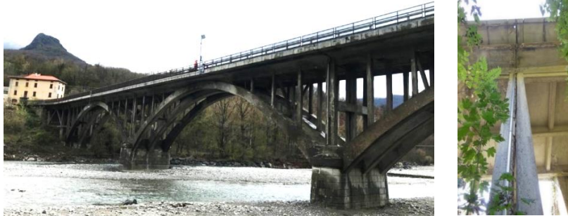
Fig. 1. Lamberti Bridge on the Ceno river (a); joint connecting two spans (b).
