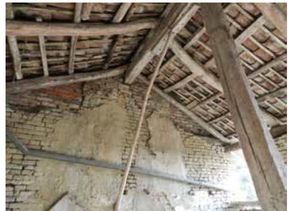
Figure 8. Wooden roof structure (credits Manuela Mattone)
