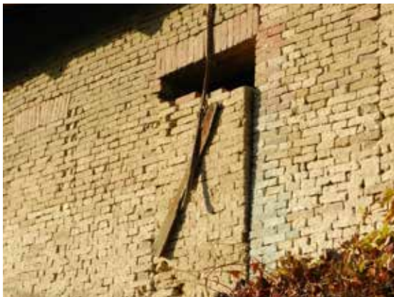
Figure 7. Brick frames surrounding the opening (credits Manuela Mattone)
