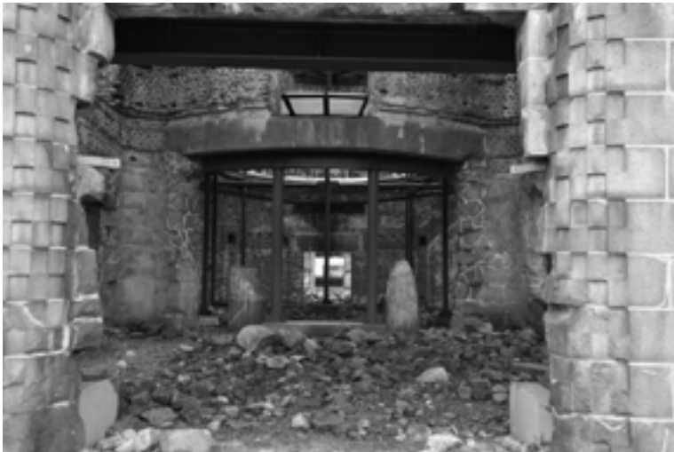
Metallic structures sustain the ruin
