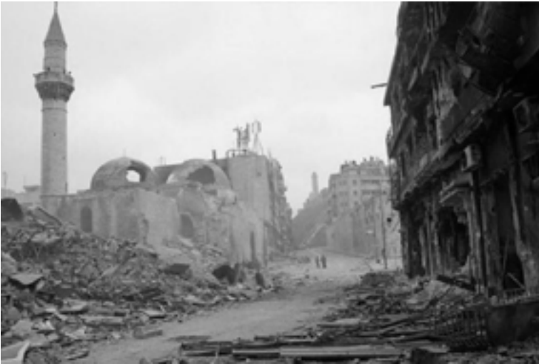
Destructions in Aleppo city, 2014
