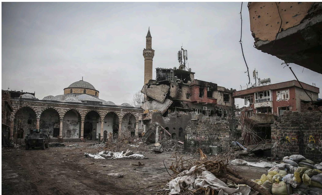
Figure 17: Damaged buildings in the Walled-City of Diyarbakir (Source: Getty Images, 2016).
