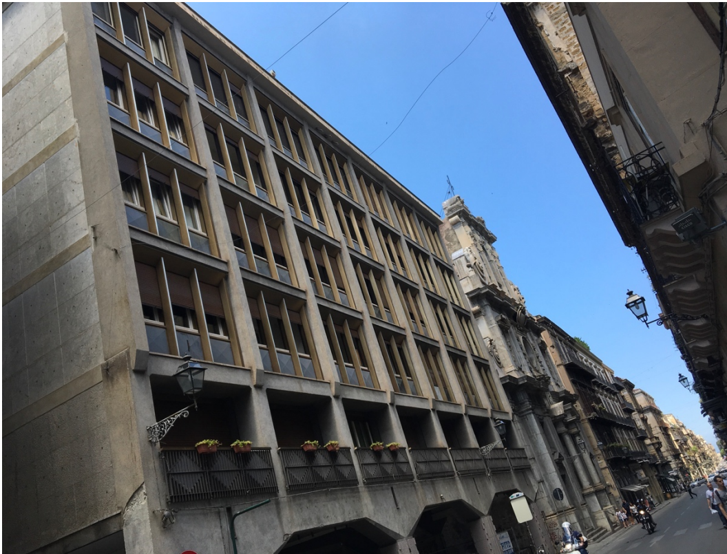
Figure 11: An example of Infill in the historical fabric (Source: Author, 2018).
