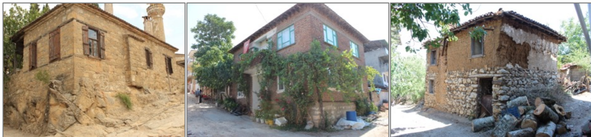
Figure 11: Diverse architectural characteristics (use of stone, brick, mudbrick, timber) in Ida Mountain (author, 2017)
