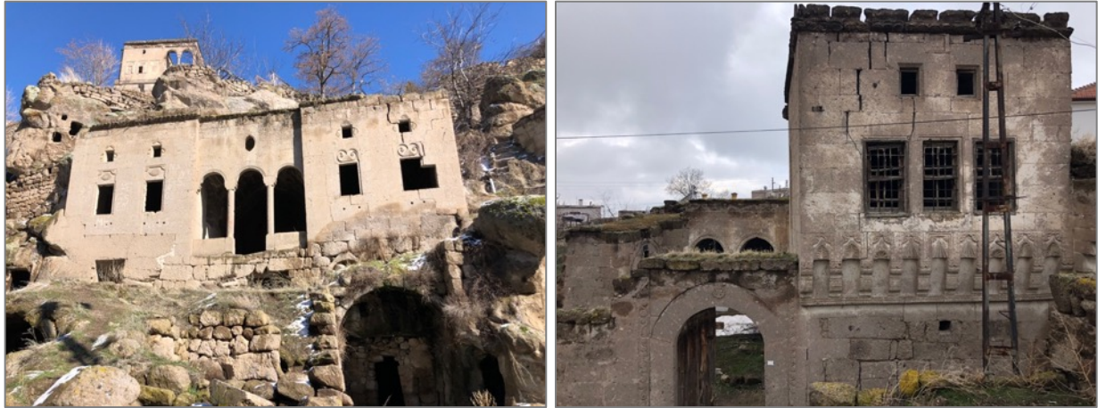
Figure 136: Structural Problems (author, 2019)
