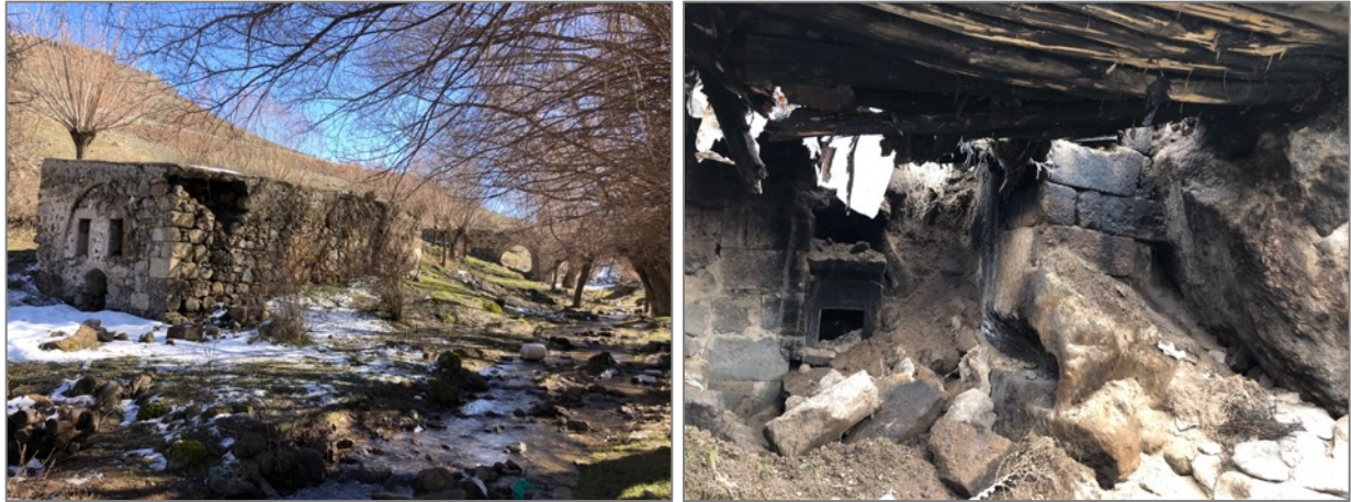
Figure 133: Demolished earth roof of the hamam and demolished furnace (author, 2019)
