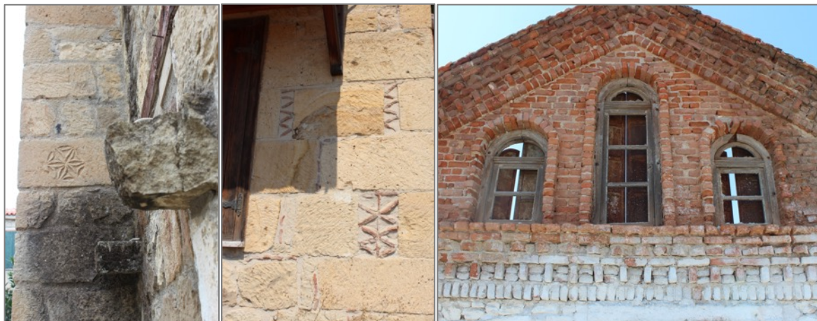
Figure 12: Architectural details and ornamentations (author, 2017)
