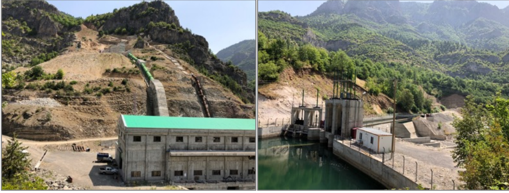
Figure 28: Construction of Hydroelectric Power Plants (author, 2018)
