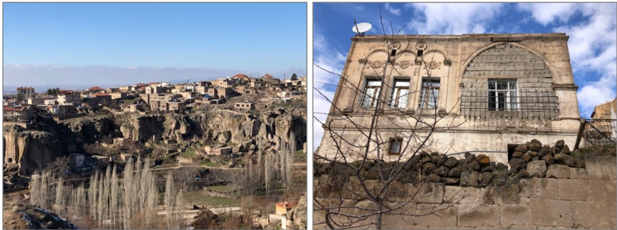
Figure 134: Inharmonious additions in the traditional settlement and improper interventions in the roof and facades (author, 2019)
