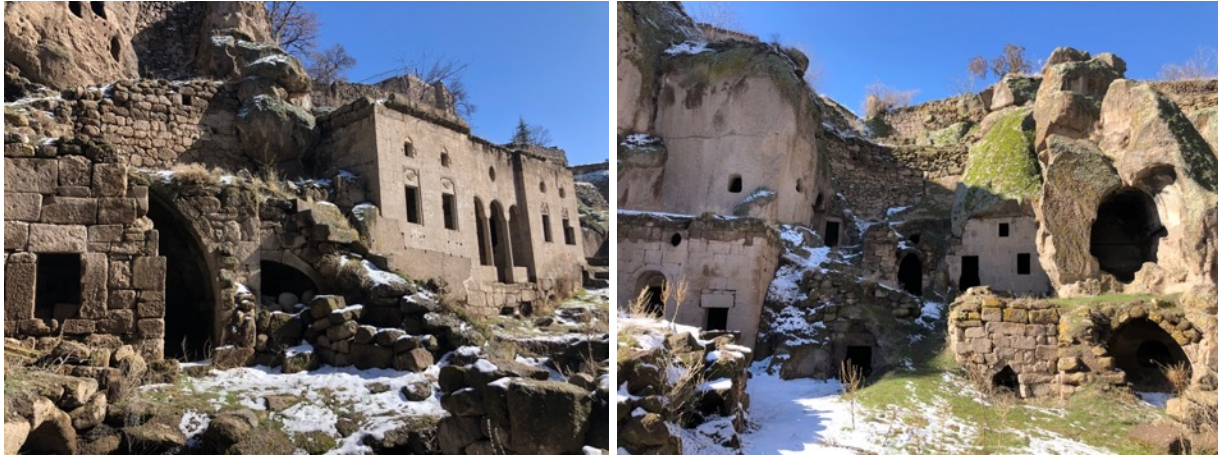
Figure 77: Abandoned places in Hengameci Street (author, 2019)
