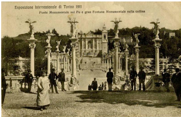
Figure 4. 1911 Postcard of the Monumental Bridge with the Courtyard of Honour and the Monumental Waterfall in the background (CDC private collection)
